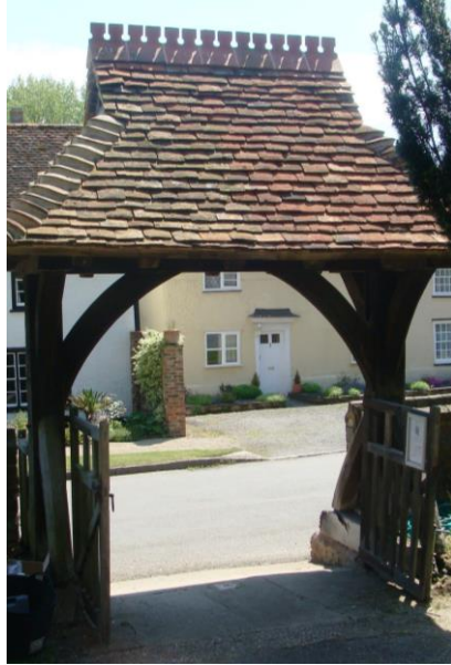
Picture 20. Recently repaired lych gate to St Mary's church.
