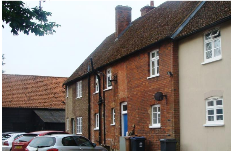
Picture 14. Residential accommodation at Westmill Bury Farm of brick construction with steeply sloping roof of historical and architectural merit worthy of retention.
