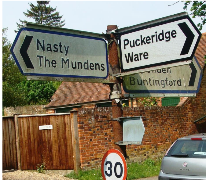
Picture 36. Directional sign post needing repainting.
