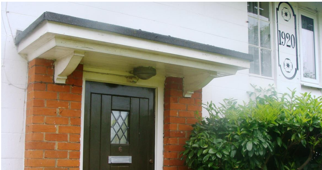
Picture 11. Unusual early 20th century council properties with original plaque and canopy detailing. Mostly original detail worthy of retention and protection.
