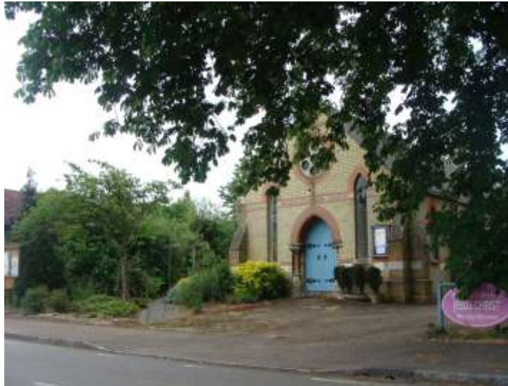
Picture 14 – Wesley Centenary Church, High Street, a fine example and representative of its type built in the late 19 th century: a potential candidate for formal listing.
