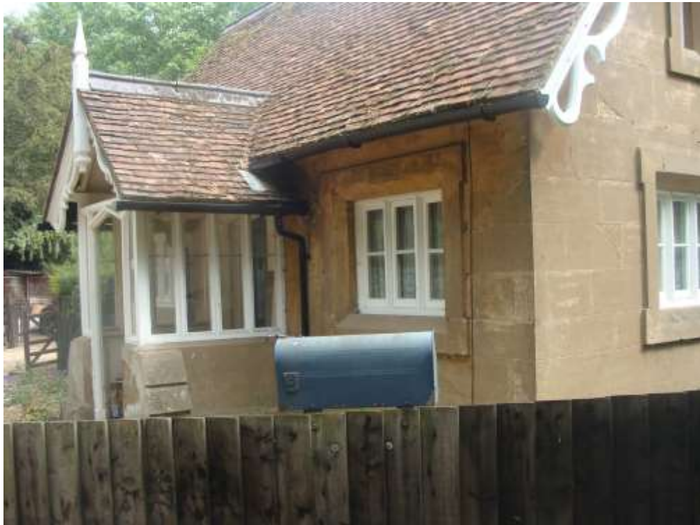
Picture 22 - Watton Lodge a delightful lodge building of ashlar facing over brick and typical Victorian barge board detailing.
