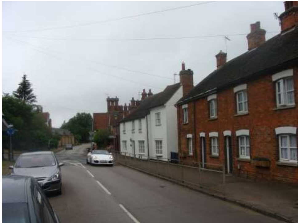
Picture 7 - High Street looking north, this part of the Conservation Area is characterised by tightly knit groups of historic buildings of quality and variety.
