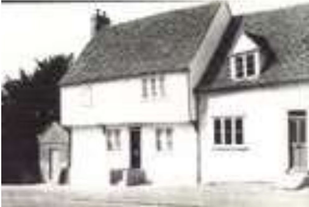
Picture 11 - The small detached building on the left of the photograph was a 19th century lock up. Its interesting and unusual former use could usefully be identified by a discreet plaque. The front entrance door is now blocked up. Photo courtesy of Mr. Alan Rattue’s local collection.
