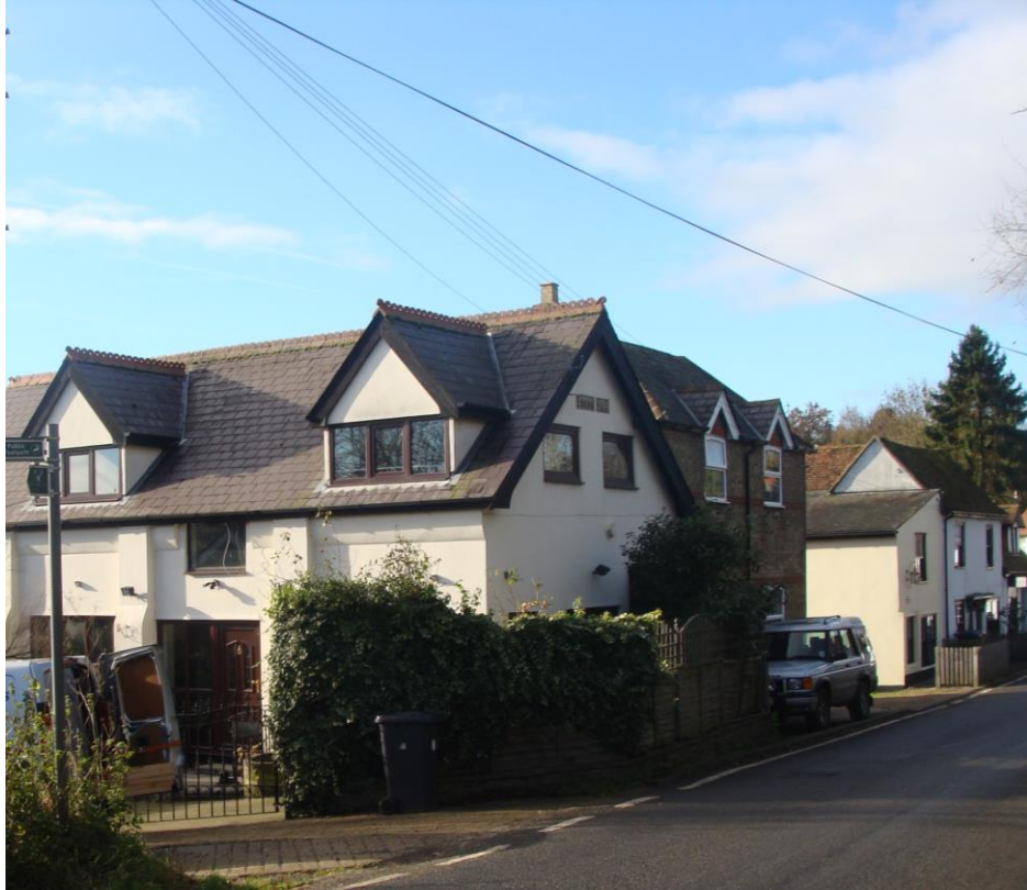
Picture 2. The former Ebenezer Temperance Hall, now altered to a degree that its original architectural and consequently historical importance is much reduced. Now rendered, entrance detail and railings removed, new dormers, new windows.
