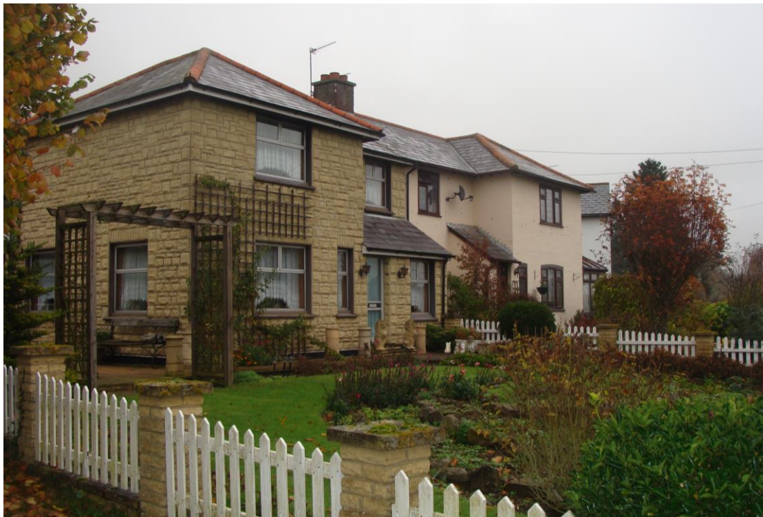
Pictures 26. The front elevations of selected properties at Hillside Cottages have been much changed and altered and are not considered to be of sufficient architectural or historic interest to remain within the Conservation Area.
