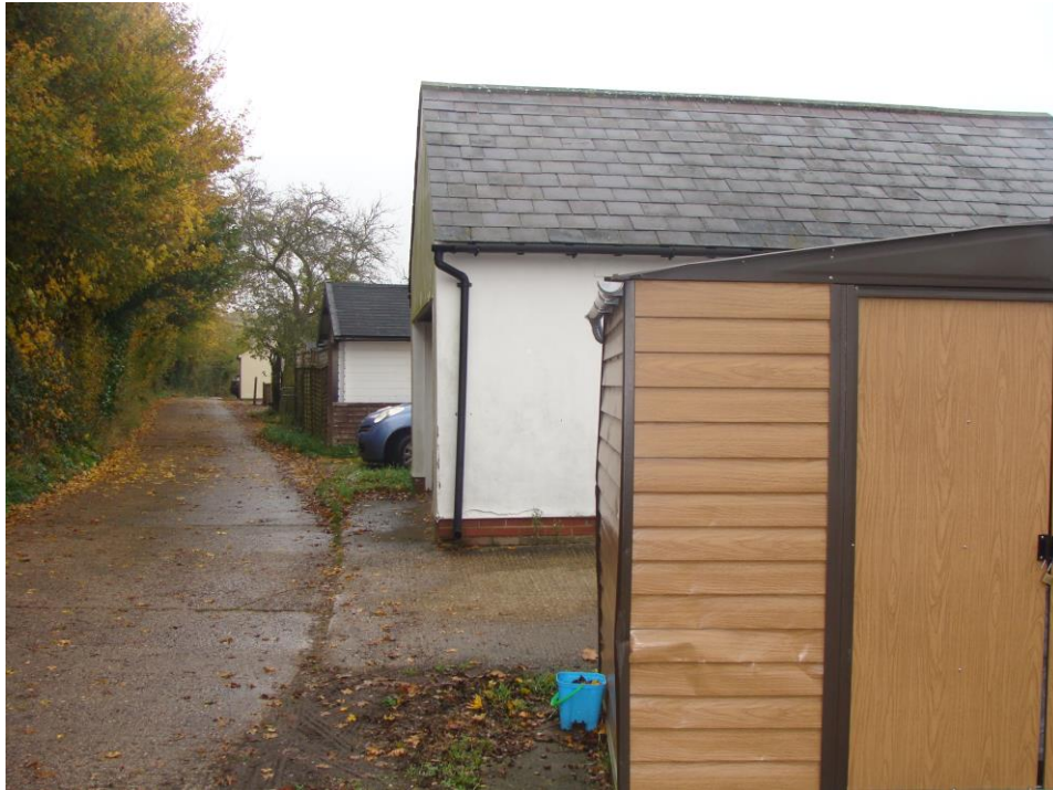
Picture 25. Miscellany of sheds, garaging, parking areas, fencing and other structures characterise the rear of Hillside Cottages.
