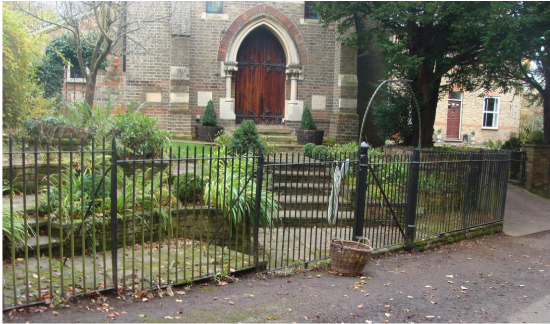
Picture 17. Simple 19 th century railings of quality to front of Wesleyan House that should be retained.
