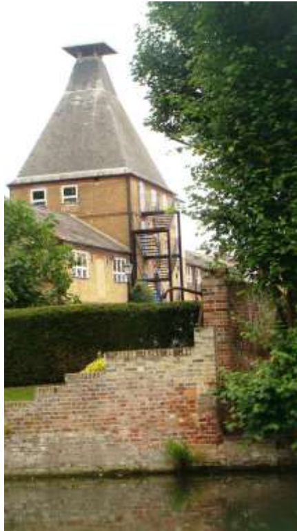
Picture 7. Prominent feature of a converted historic building prominent in the townscape. It is very important that the limited number of such symbols of Ware's past are retained.
