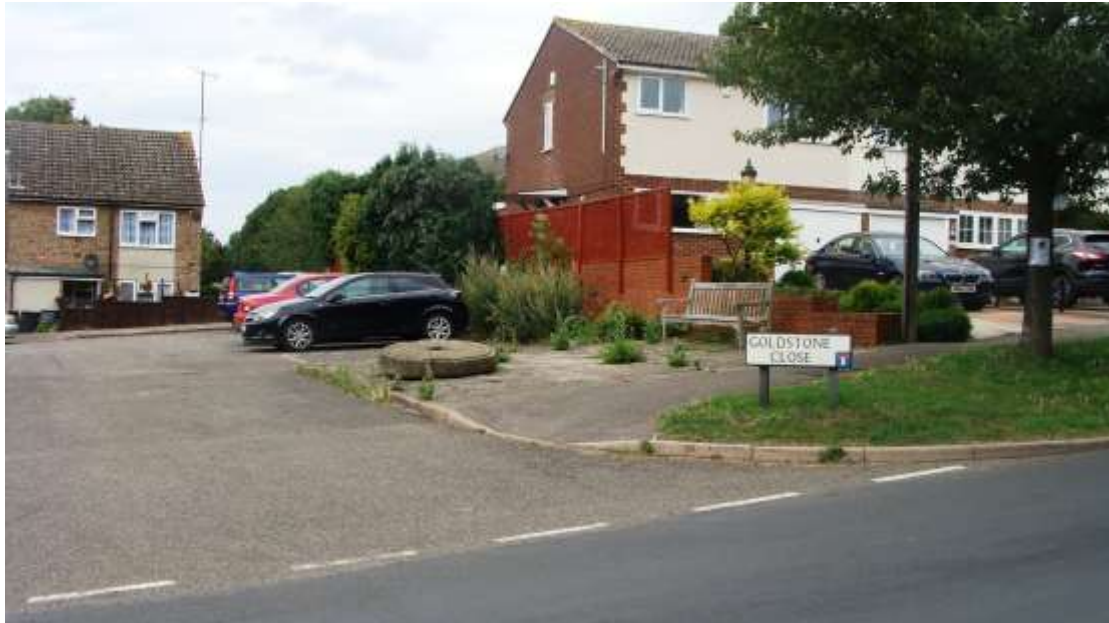
Picture 98. Communal sitting area at Goldstone Close in real need of improvement.
