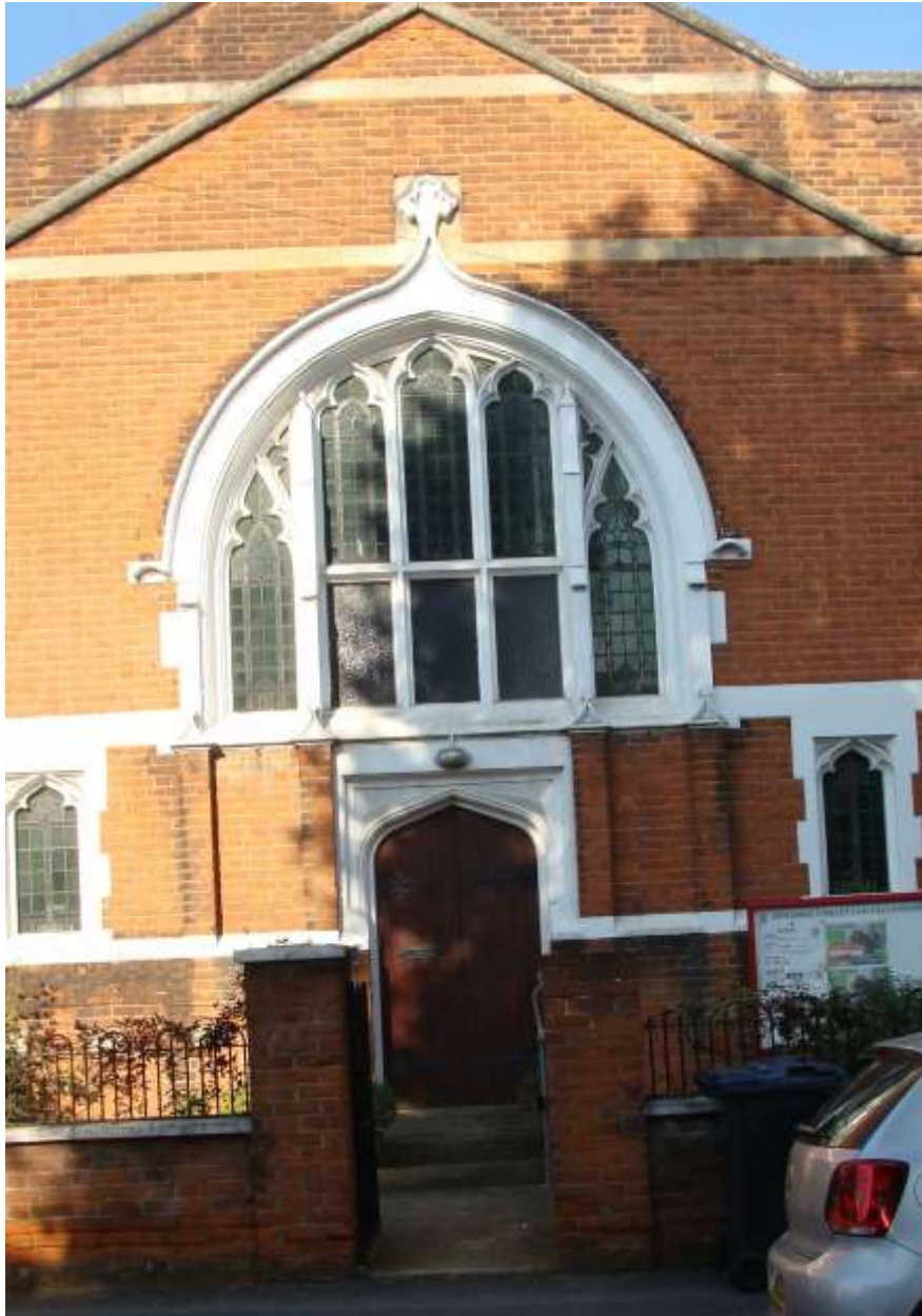
Picture 83-84. Springs Christian Fellowship building south end of New Street. It makes a significant contribution to the street scene. Upper picture shows interesting inscribed brick.
