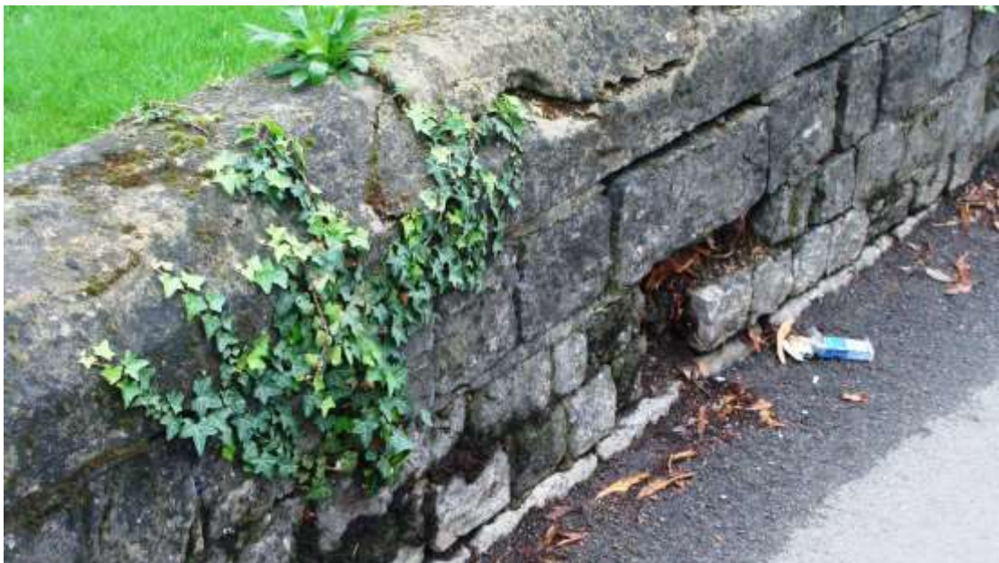
Picture 61. Mid 19th century boundary wall to Christ Church in need of repair.
