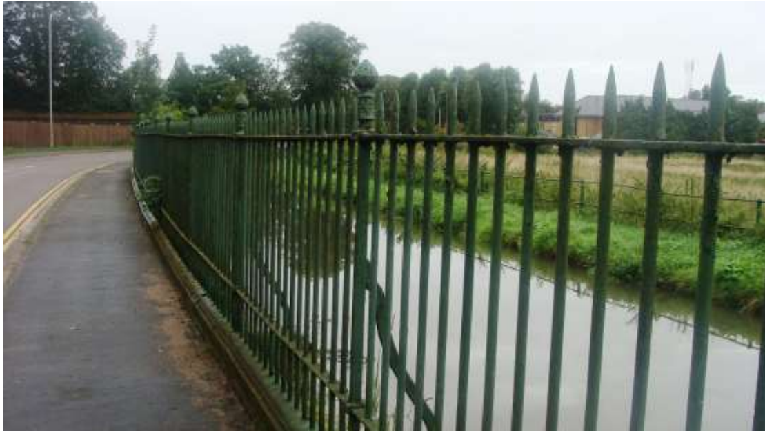
Picture 43. Fine listed railings believed to be owned by Thames Water which make a very positive contribution to this part of the Conservation Area.
