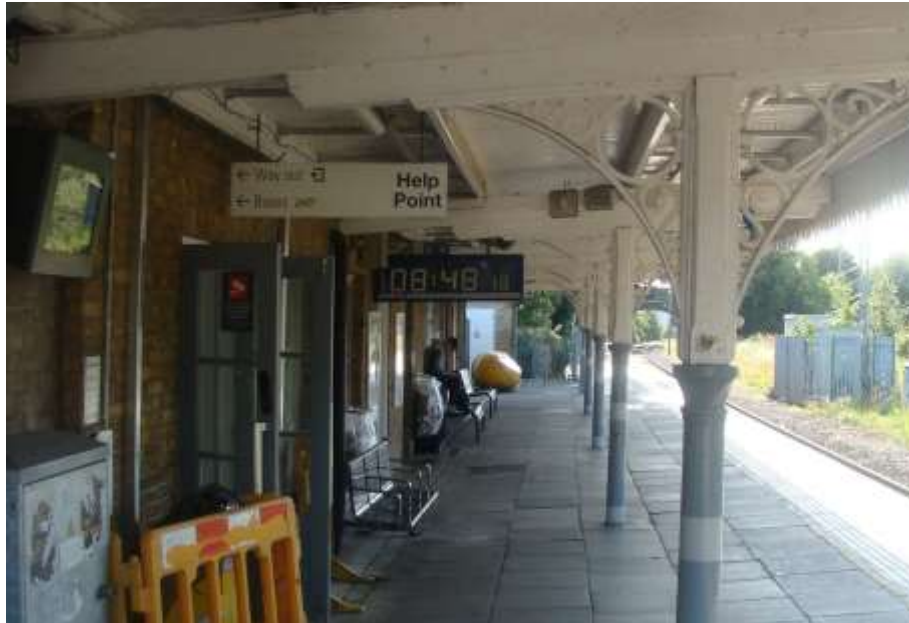
Picture 50. 19th century station part of the industrial heritage of the town. Canopy and cast iron supports are typical.
