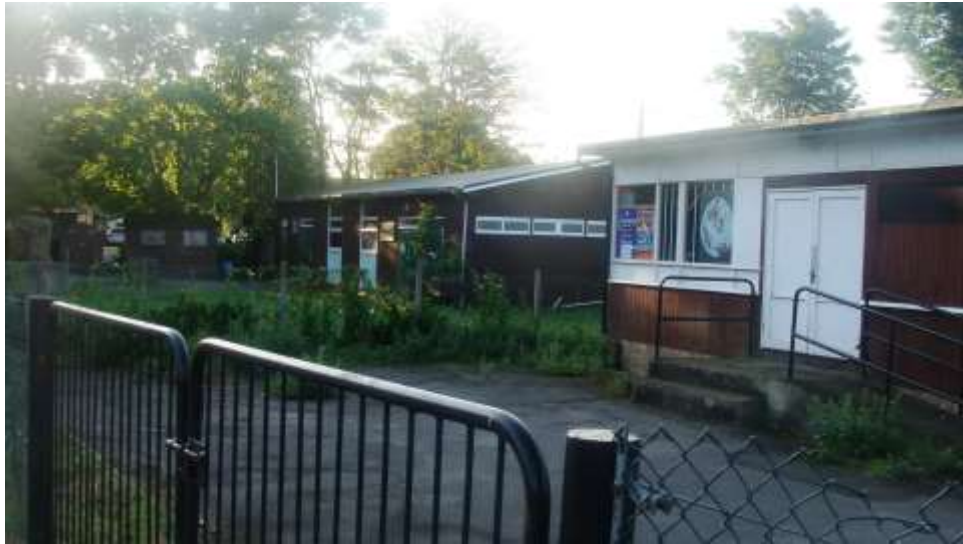
Picture 55. Prefabricated buildings (Scouts and Air Training Corps) Broadmeads. This site detracts from the quality of the Conservation Area and needs improvement.
