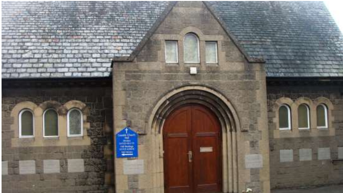
Picture 19. Leaside Church Hall a good quality building of its type.
