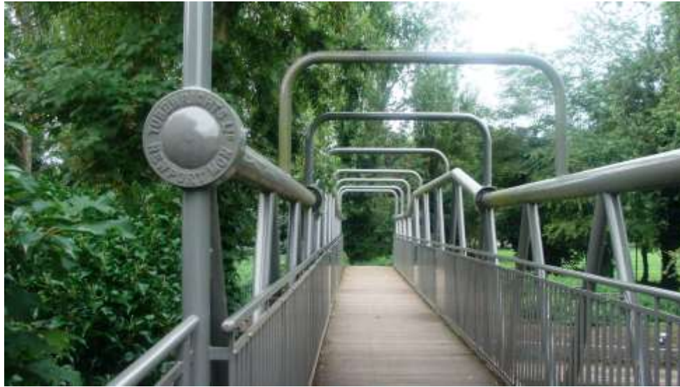
Picture 32. Fine contemporary footbridge. Modern architectural solutions certainly can be appropriate in an historic location.
