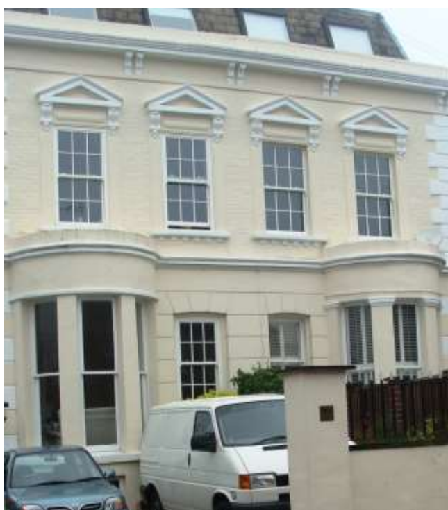
Picture 79. Nos. 105a- 105b New Road. A finely detailed building that makes a significant visual contribution to the street scene.
