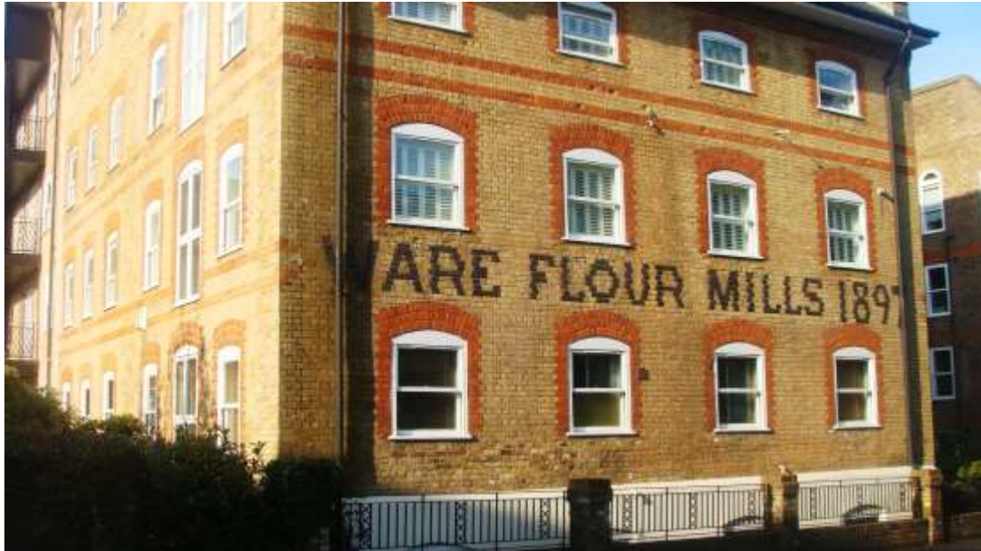
Picture 40. Successful conversion of non listed Ware Flour Mills buildings corner of Amwell End and Viaduct Road. The visual impact of modern window detailing is limited and works relatively well because of its repetitive design.
