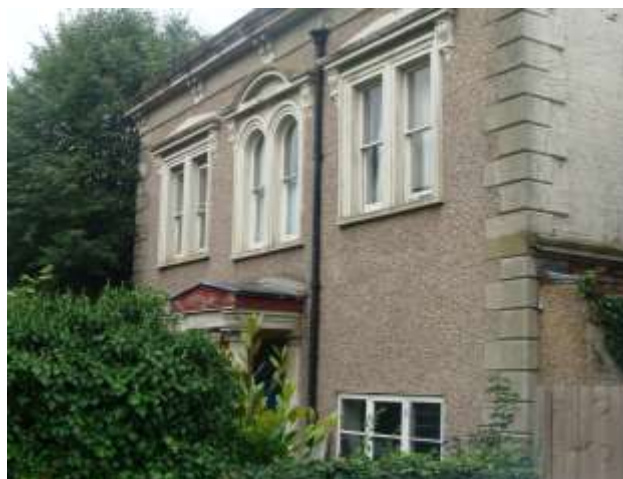
Picture 78. Fine architecture detailing no. 95 New Road.
