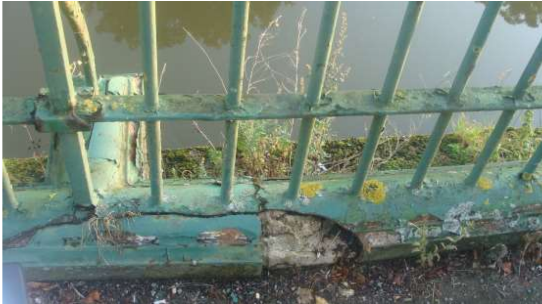
Picture 44. Detail of railings some of which are in need of repair and or repainting. In some areas removal of self set sycamores would be beneficial.
