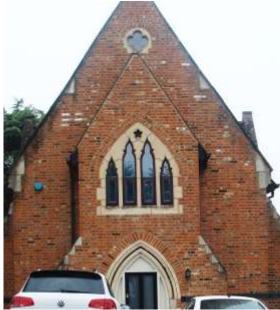
Picture 74. No. 48 New Road - Former chapel now in residential use.
