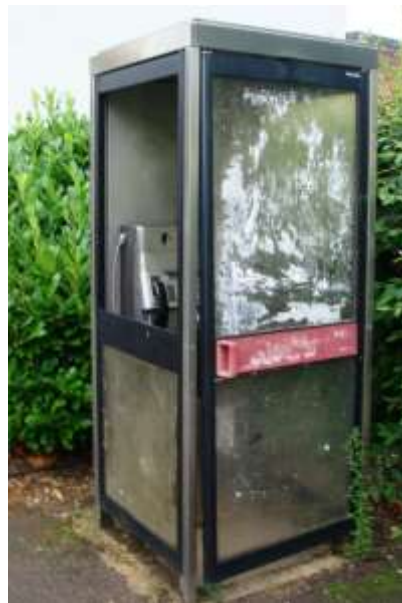
Picture 39. Modern 20th century telephone kiosk, vandalised and in poor condition. Its repair or removal if no longer in active use recommended.
