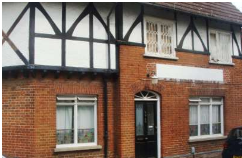
Picture 108. No. 46 Priory Street, interesting late 19th century building.
