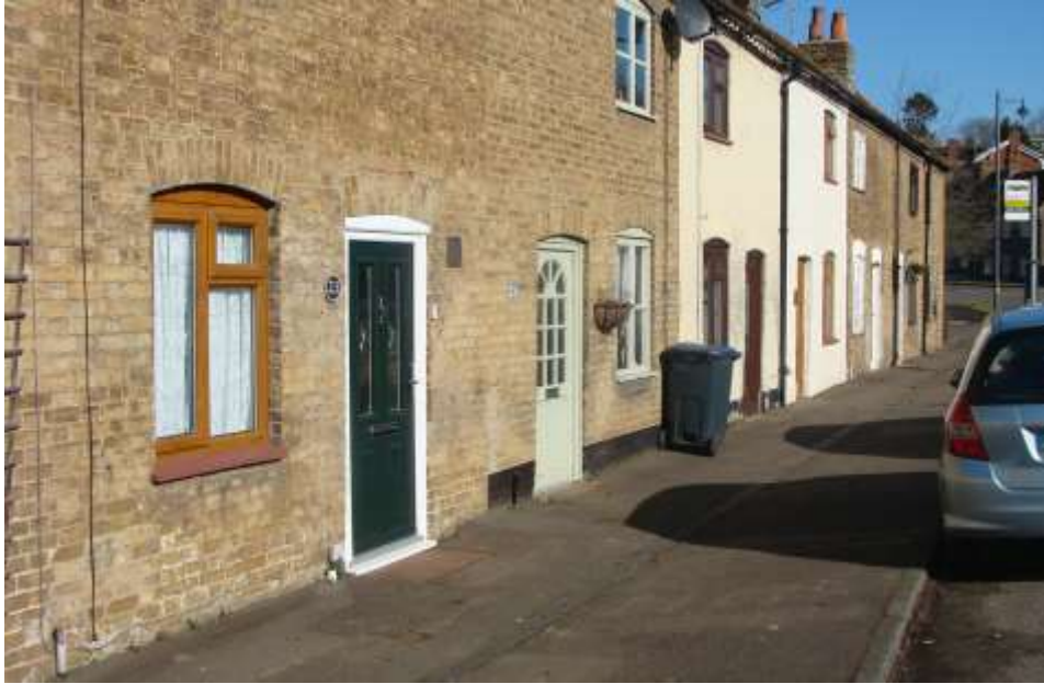
Picture 3. 20-29 Cambridge Road. Terrace of Listed Buildings dating from late 18th century. Whilst doors and windows are in original openings, a more pleasing result would have been achieved had common designs been applied (see picture below).
