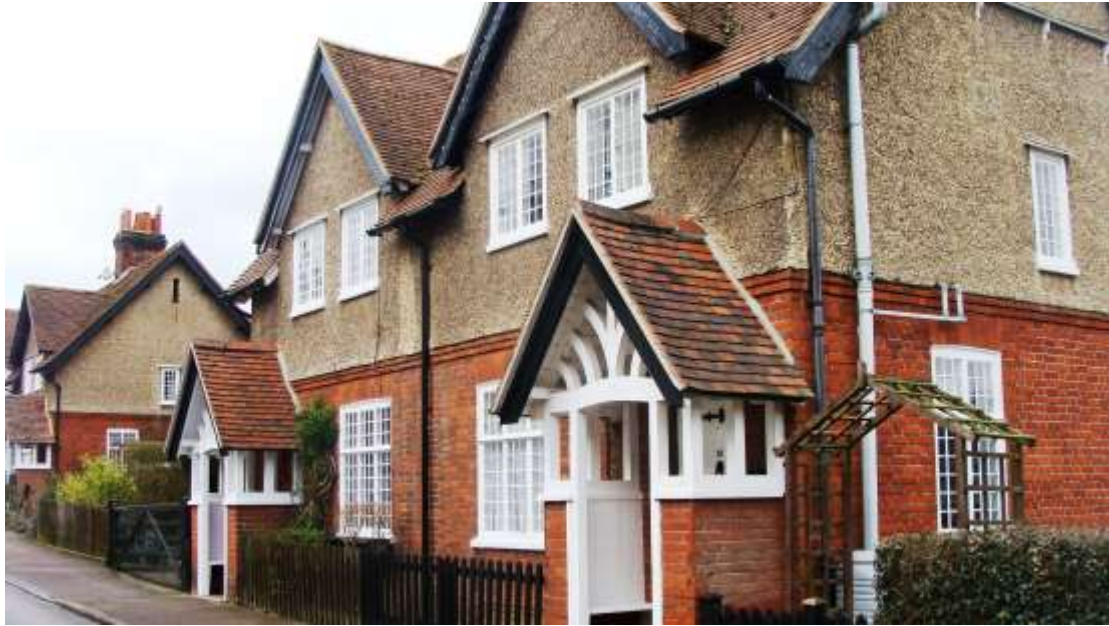
Picture 9. 11-13 Ermine Street - fine late 19th/early 20th century cottages with much original detailing.
