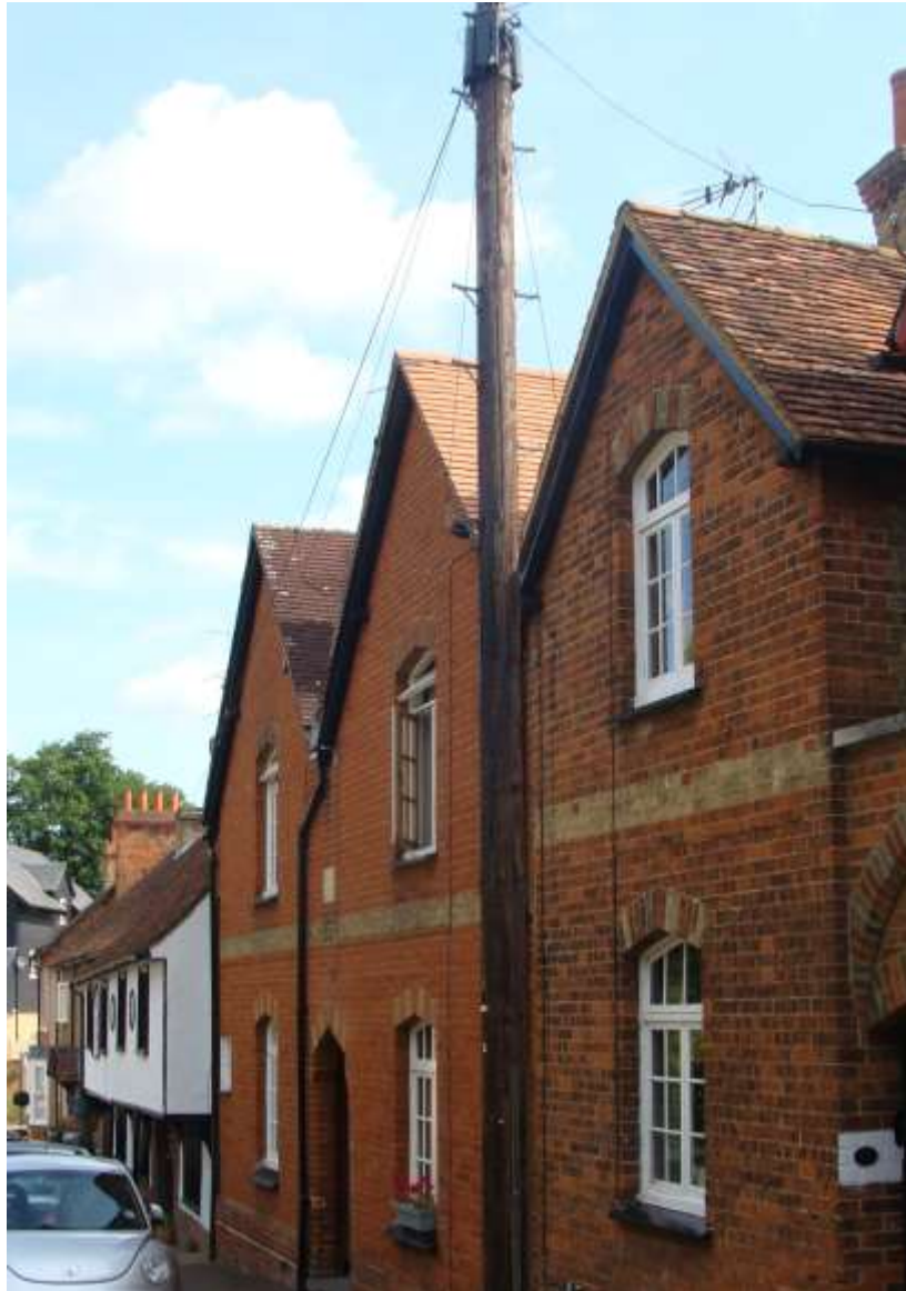
Picture 25. Utility poles detract from the high quality of the Conservation Area in this location on Ermine Street. The potential of resolving the situation could be explored with the utility company.
