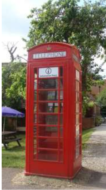
Picture 19. K6 Telephone kiosk, well maintained and in good condition, now an information point.
