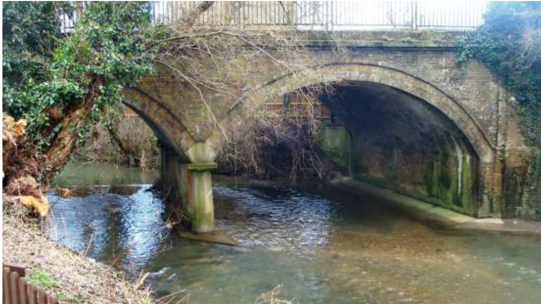
Picture 5. Listed road bridge over River Rib. Considered to be very fine in some of its detailing.
