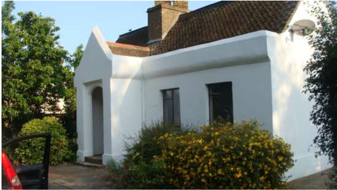
Picture 8. South Lodge - single storey rendered Lodge, tiled roof slate ridge and later metal windows. Whatever its status in law (i.e. curtilage listed or not) it is a building that is worthy of retention.
