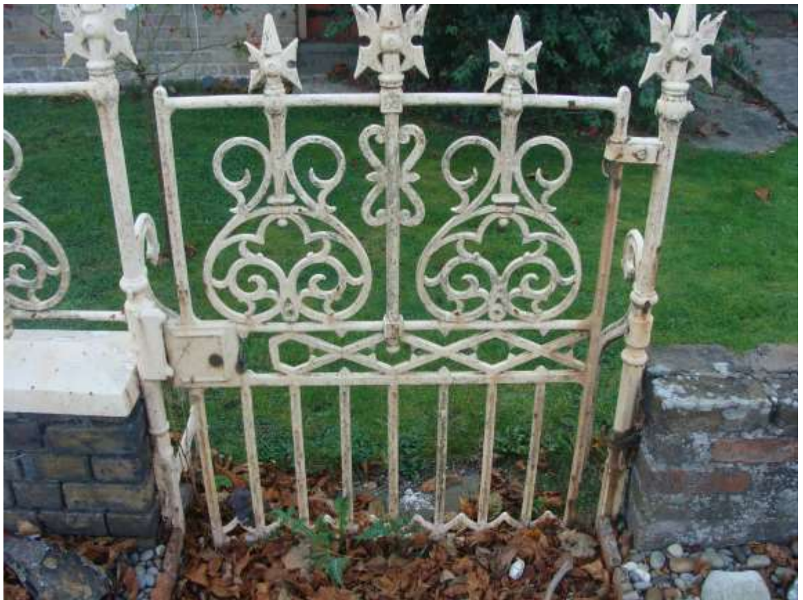
Picture 17 – Decorative 19 th century metal gates and fencing to Warrax Cottages.
