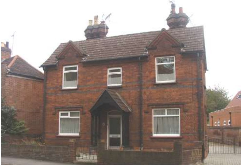
Picture 29 – 19 th century building of pleasing mass and proportion has been compromised by modern windows that are unsympathetic.
