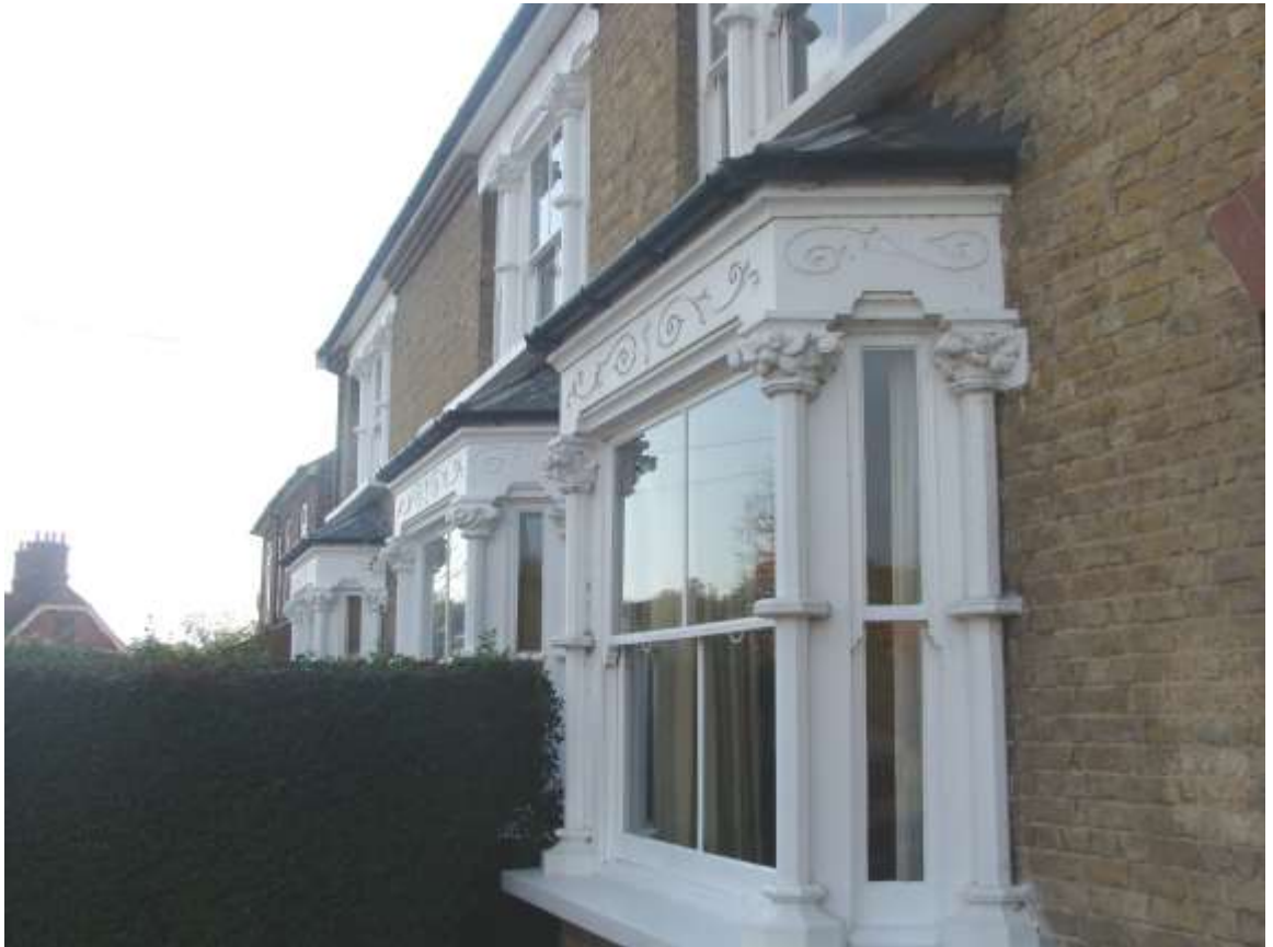
Picture 14 – Unaltered late 19 th / early 20 th century decorative architectural detailing to nos. 130-132 Cappell Lane, particularly worthy of protection.
