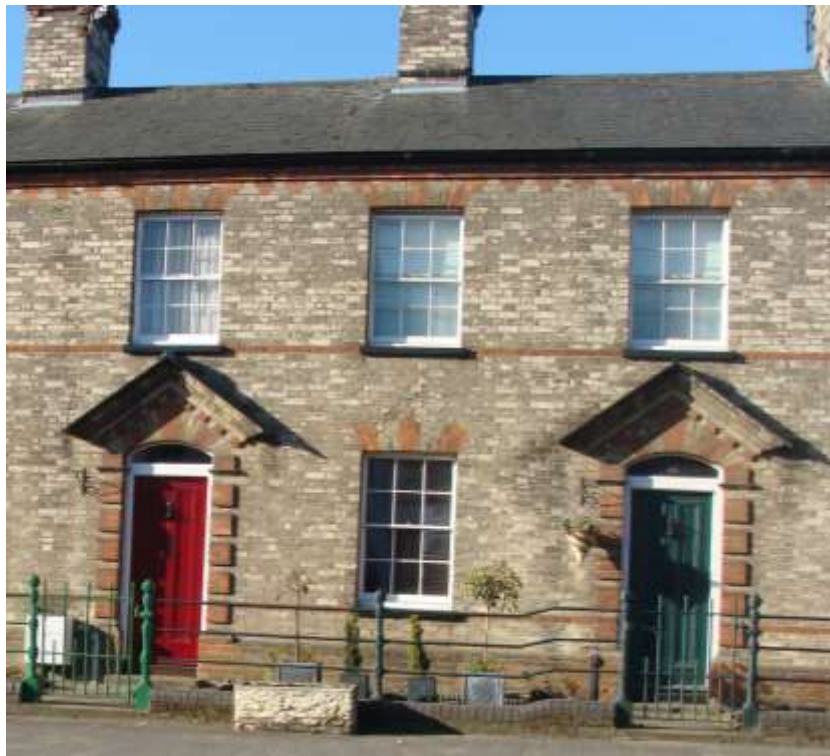
Picture 29a – building elsewhere of similar date with pleasing repetitive window detailing.
