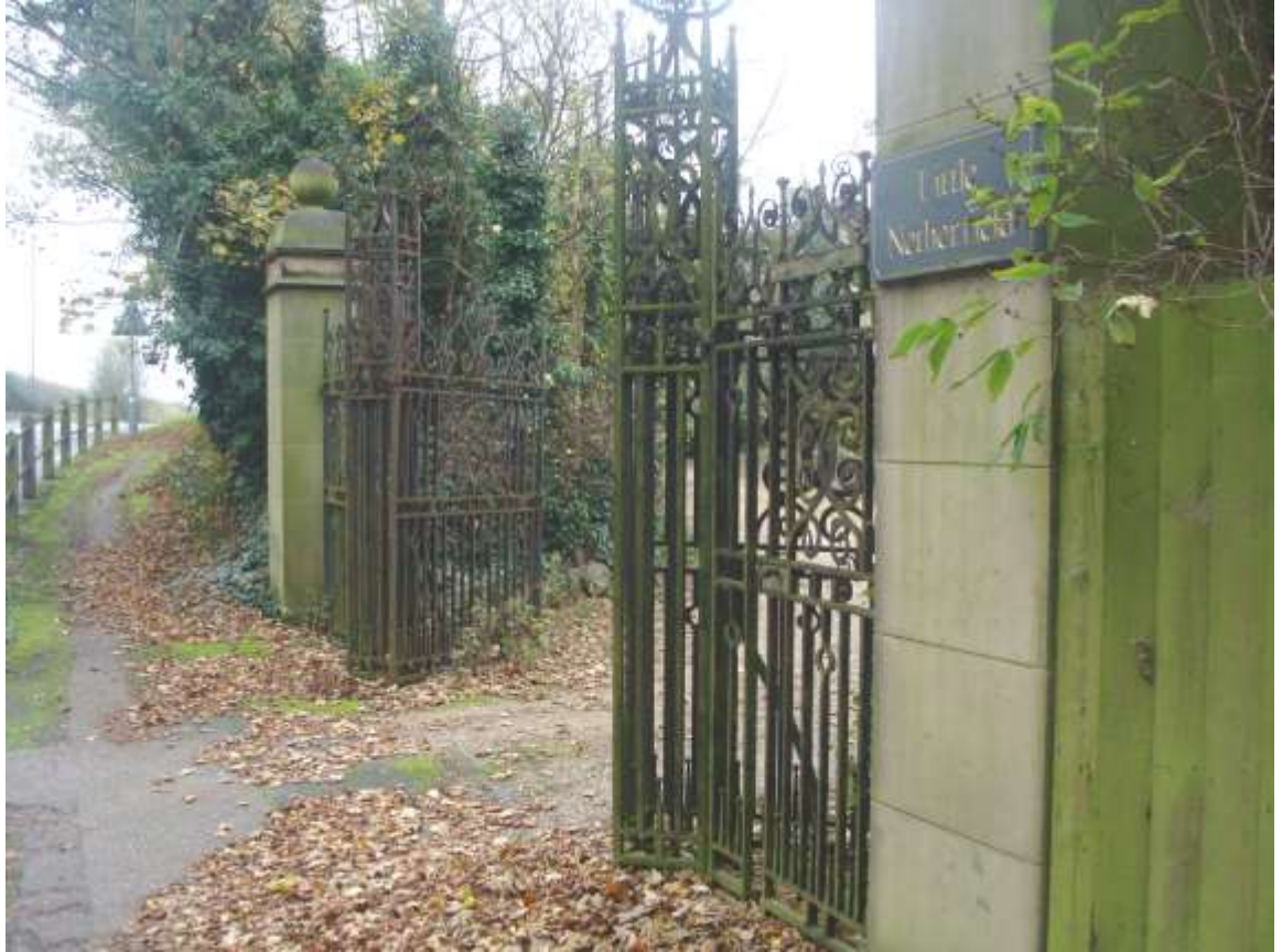
Picture 19 – 19 th century listed gates and piers formerly to Netherfield House, Cats Hill.
