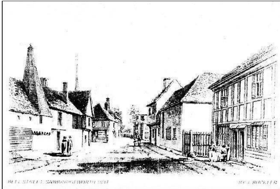
Sketch of Bell Street in 1834 up to the junction with Knight Street The Market House is on the left at the former (Buckler 1834: Beams Collection)
