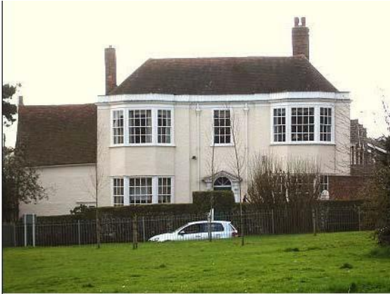
123 Sheering Mill Lane
