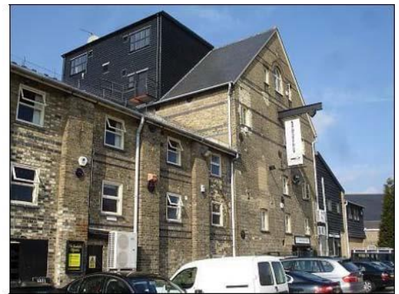
The West Maltings from within the site, Station Road
