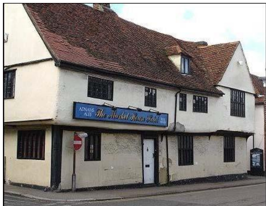
The Market House Hotel, 42 Knight Street
