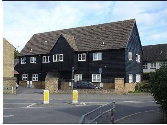
Weatherboarded barn, Station Road, formerly part of Walnut Tree Farm, Cambridge Road
