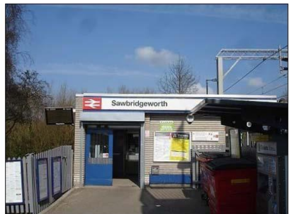
Sawbridgeworth Railway Station, Station Road
