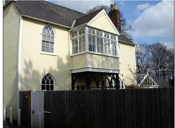
136 Sheering Mill Lane
