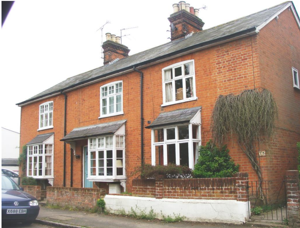
Picture 5 - Nos. 11-15 Buntingford Road, late 19 th /early 20 th century, non listed properties of quality.
