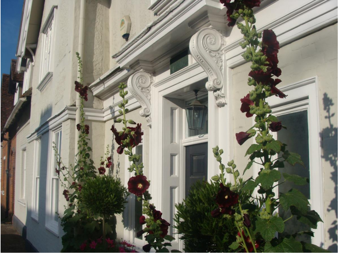
Picture 6- The importance of fine architectural detailing.
