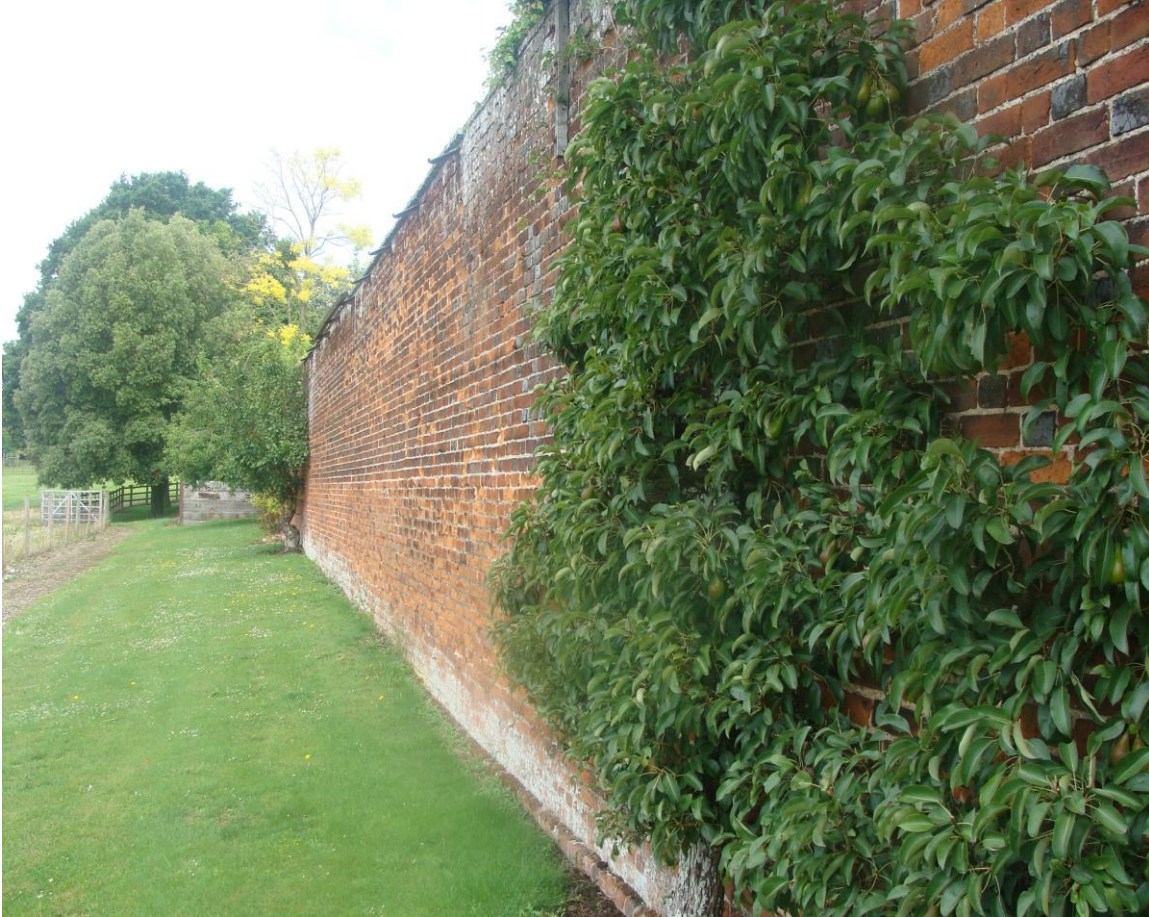
Picture 44- Distinctive wall approximately 4 m in height, remnants of 19 th century tension bolts and fittings for training fruit trees observed.
