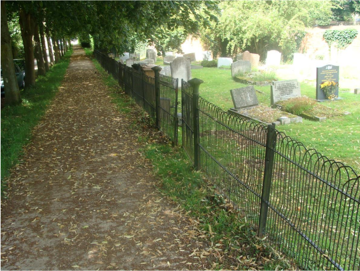
Picture 15- Simple and delicate early/mid 20 th century railings enclosing churchyard extension. The avenue of trees adjacent is an important feature and one that is repeated elsewhere in Much Hadham's streetscape.
