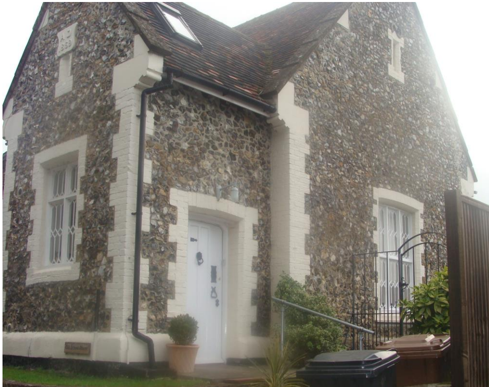
Picture 18- Old School House, Tower Hill. Formerly a 19 th century Infants School and typical of its type; a possible candidate for formal listing.
