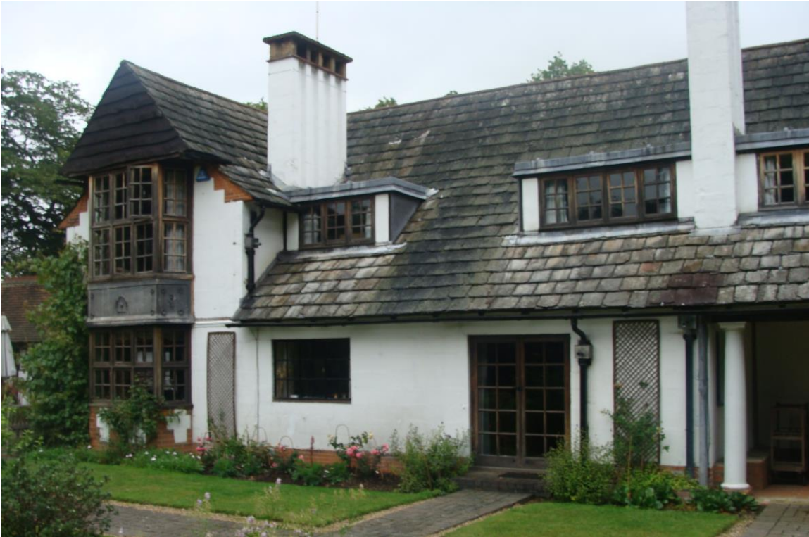
Picture 30- Daneswood, an unusual 20 th century Listed Building built in the Arts and Crafts style with distinctive Westmoreland slate roof.
