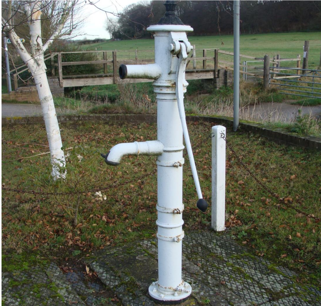
Picture 5 - A fine 19 th century pump of considerable artistic, social and technological interest. Several of the blue brick pavements need re-setting.
