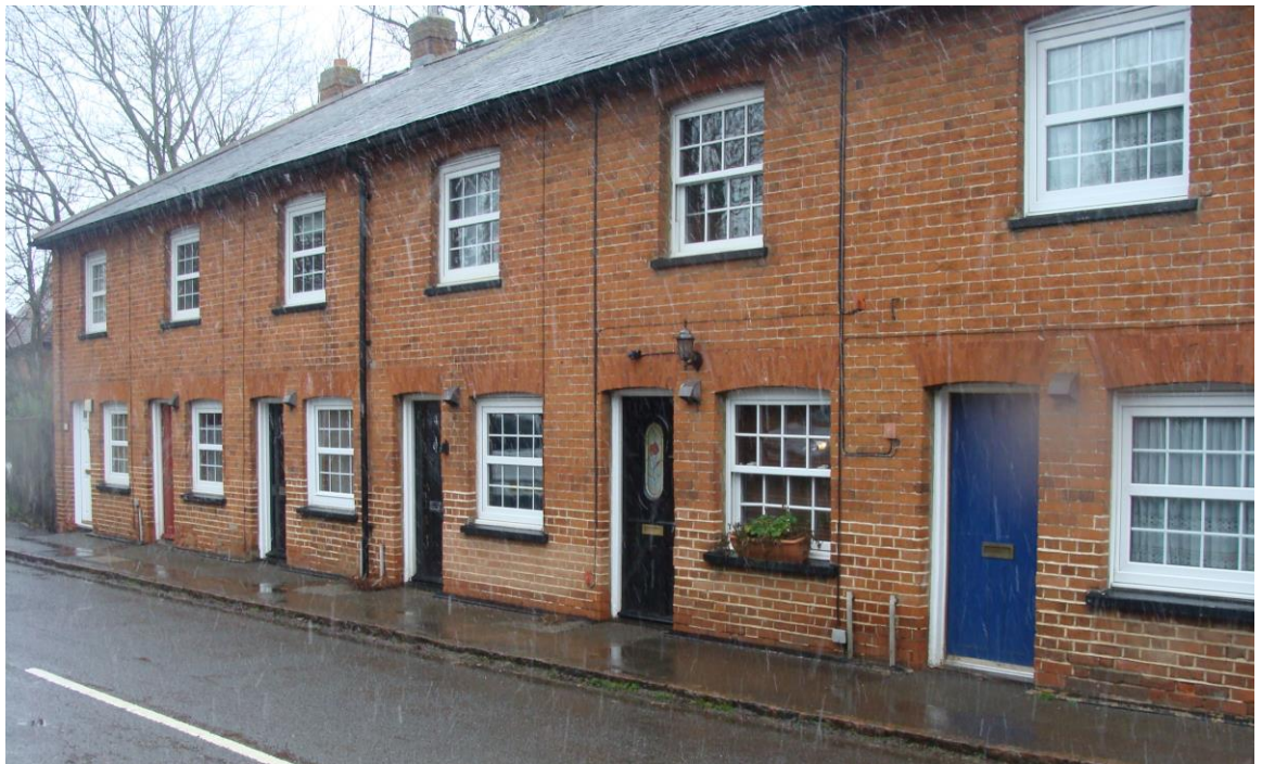
Picture 12 - Red Brick Cottages. Windows are modern replacements but because they are all similar they achieve an acceptable degree of architectural rhythm and unity.
