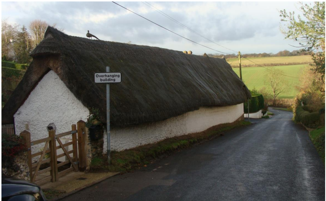
Picture 7 – Thatched building with clay lump walls at Ford Hill. It survives as an obsolete form of building construction of great interest.
