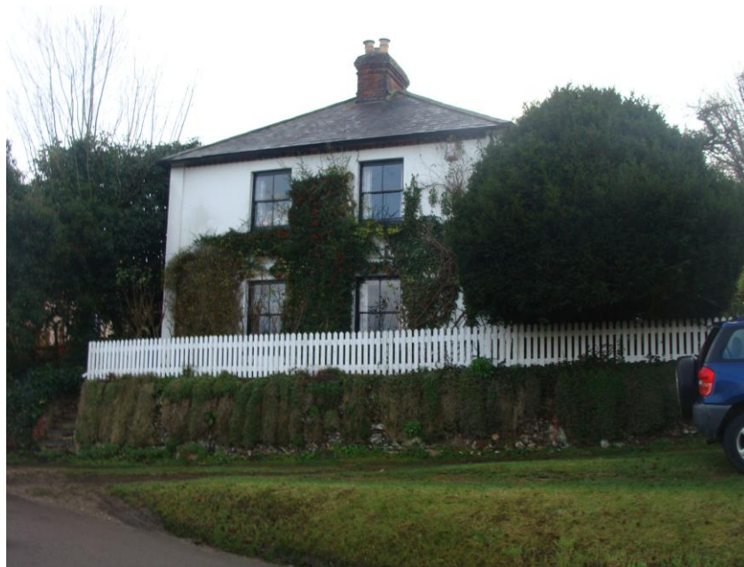
Picture 10- The Manse, a late 19 th century unlisted prominent house on elevated position with pyramidal slate roof.
