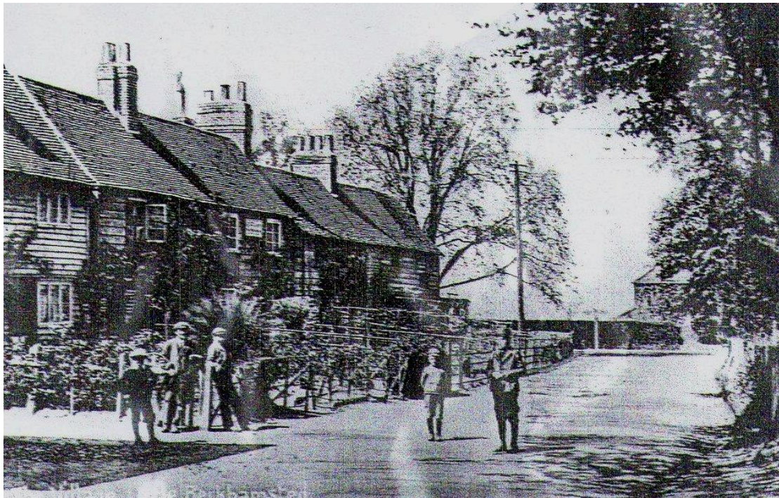
Picture 1. Looking north along Church Road towards the location of the War Memorial. The latter was erected in 1921 so this photograph must have been taken before that date. Reproduced courtesy of Hertfordshire Records and Local Studies.
