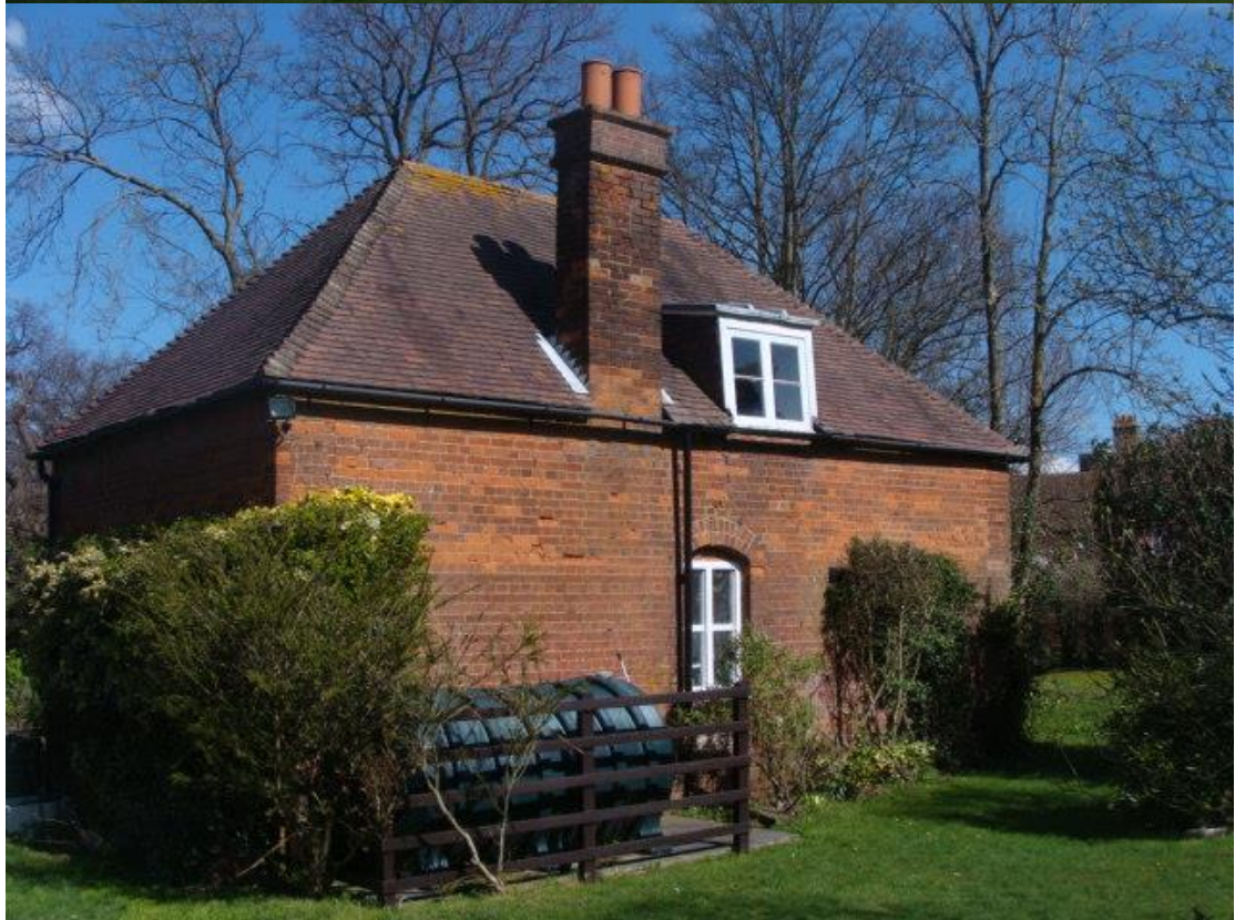
Picture 13. Trewinnard and outbuilding being formerly the Vicarage. A handsome building most worthy of retention with a number of high quality architectural features. The owner advises windows to front elevation are like for like replacements which represents best conservation practice.
