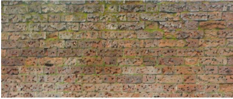
Picture 28 and 29. Detail of fine walled garden to north of Garden House. The decorative wooden gate is now bricked up behind. It previously provided access through to Culverwood House. Note central statue and remains of iron arches. Lower picture shows wall pockmarked by supports for fruit trees whose branches were pinned to the brickwork.
