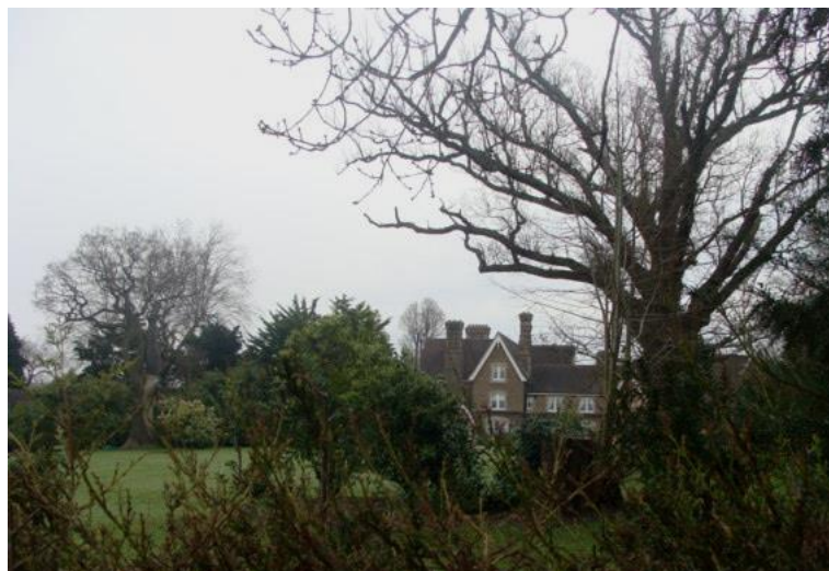
Picture 17. Culverwood House viewed from the public domain.
