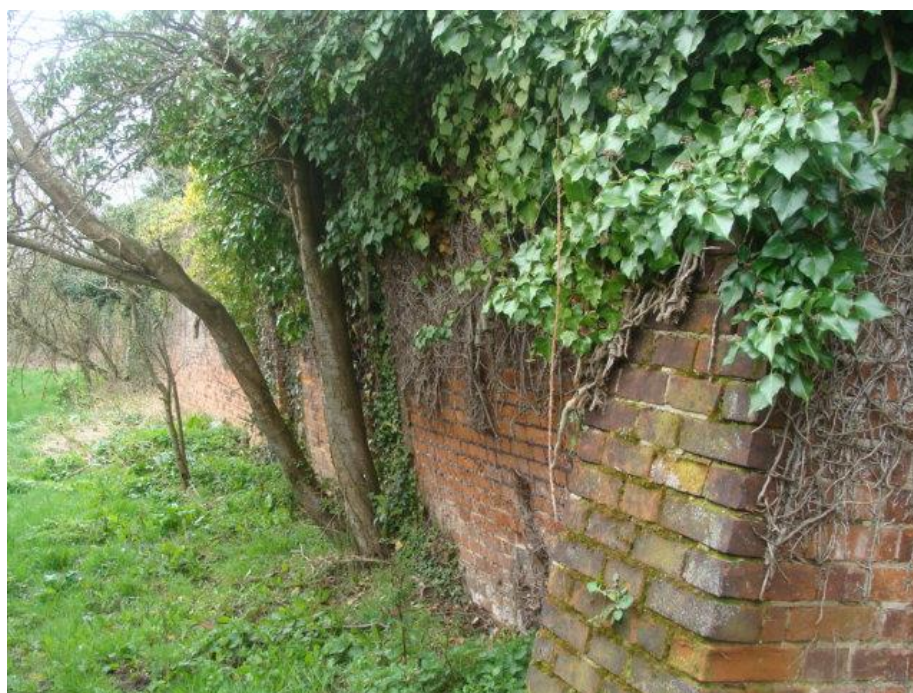
Picture 23 - Detail of fine walls to walled garden historically associated with Danes. They are generally in good condition but would benefit from removal of selected vegetation in some locations such as ivy that may be causing damage.
