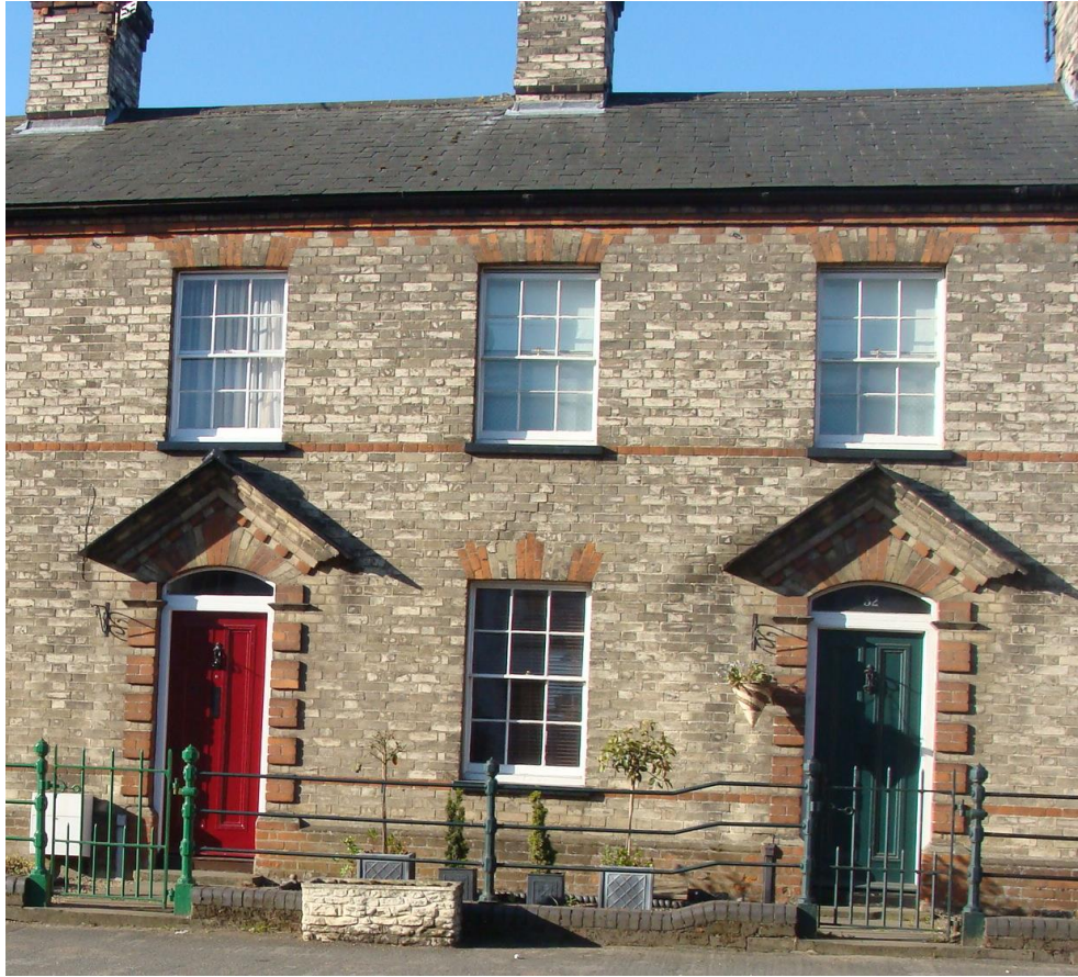
Picture 7 – A terrace not local to Hunsdon: the purpose of this photo is to illustrate the importance of design detail. The successful character of historic terraces in part depends on simple repetitive detailing, including doors. Expression of ownership can be provided by painting doors different colours.
