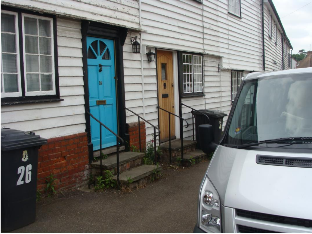
Picture 6 - White weatherboarding is an important architectural feature of some Listed Buildings in Hunsdon.
