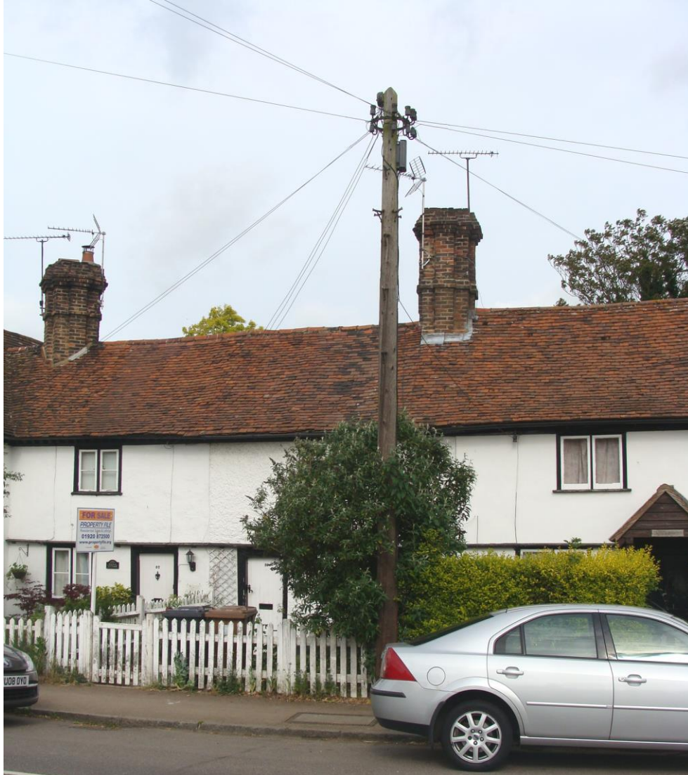
Picture 12 – One of several utility poles that detract from the high visual and historic qualities of the Conservation Area.
