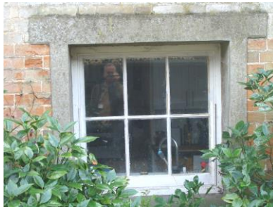
Pictures 15-18. Yew Lodge and Grange Lodge, prominent in the street scene with selected details worthy of additional protection.
