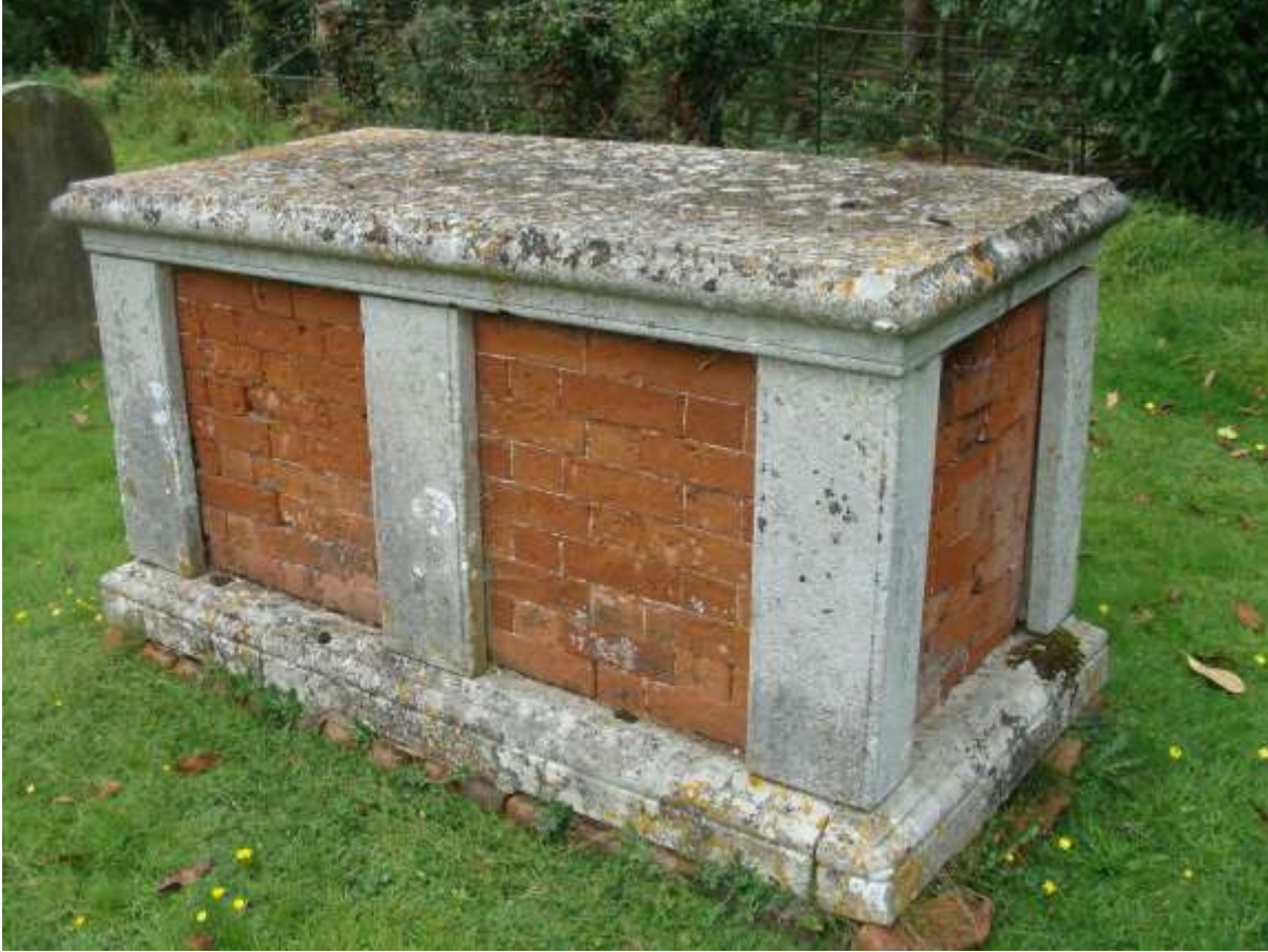
Picture 13 – One of many fine chest tombs in the churchyard, this one being of stone and rubbed brick.
