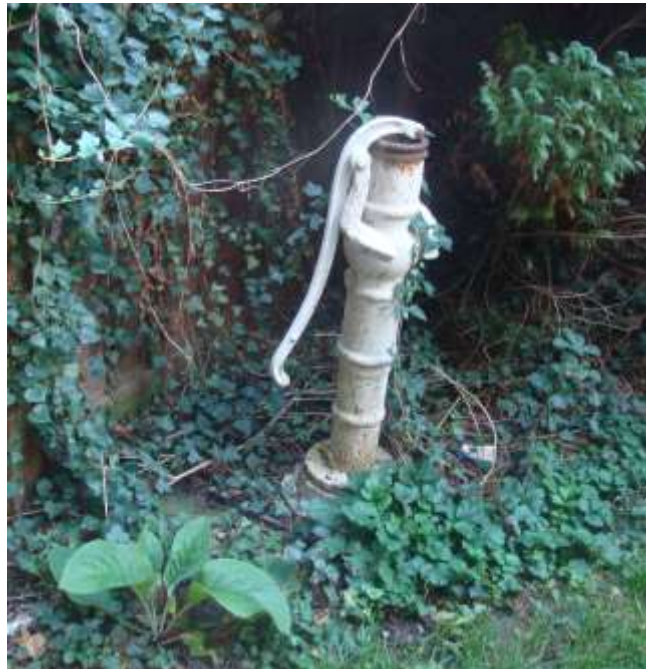
Picture 17 - 19 th century pump to rear of Prince of Wales PH in urgent need of restoration.
