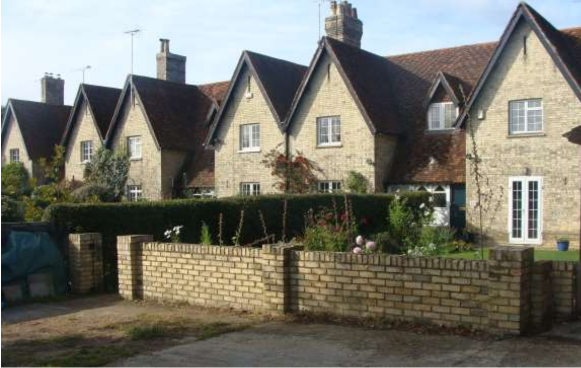
Picture 10 - Nos. 260 – 274 Hertingfordbury Road, an unlisted 19 th century terrace whose imposing mass contributes to the Conservation Area in this location.
