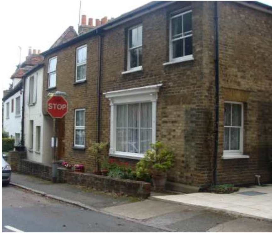
Picture 8 - No. 267 Hertingfordbury Road and nos. 1- 3 St. Mary's Lane. Unlisted buildings whose mass and selected architectural details contribute to the quality of the street scene.
