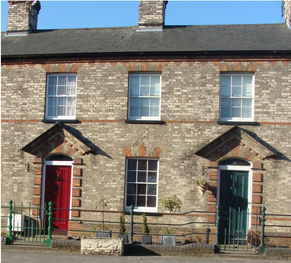
Picture 17. A listed terrace not local to East Hertfordshire. The purpose of this picture is to illustrate the importance of design detail in relation to traditional late19th/early20th century terraces. There are large numbers of similar unlisted terraces in Hertford identified by this appraisal as being important. Retaining the character of such terraces in part depends on keeping simple original repetitive detailing, including doors. Compare this simple solution with some of the previous illustrations which do not provide any sense of architectural 'rhythm' and are disruptive. Expression of ownership can be provided by painting doors different colours.
