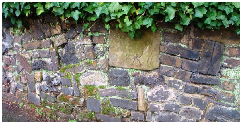
Picture 87. Interesting wall of random construction.
