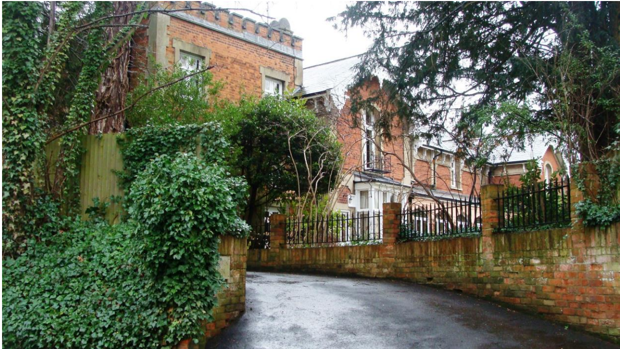
Picture 50. The important grade II* Listed Building, Warren Park.
