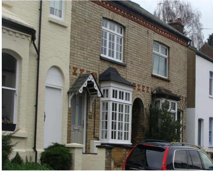
Picture 4. Another similar example, various replacement window types.
