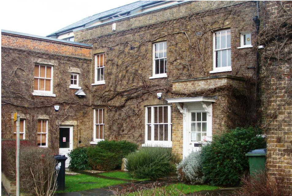
Picture 110. Handsome building corner Railway/Priory Street; most worthy of retention.
