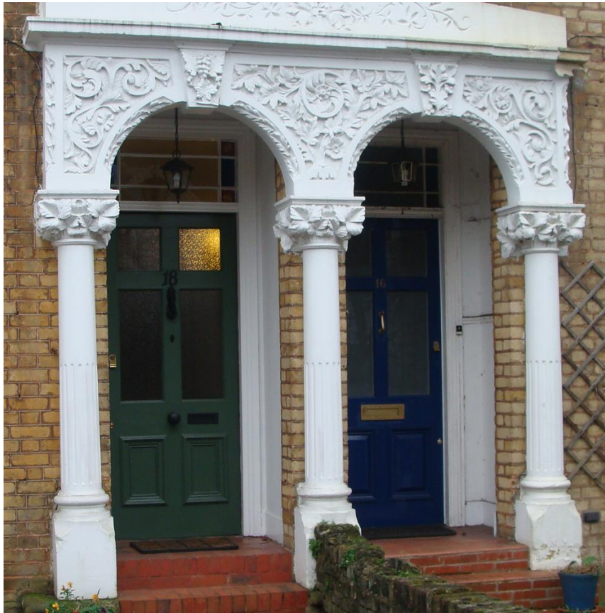
Picture 135. Highly decorative late 19th century detailing to properties west side of Queens Road.
