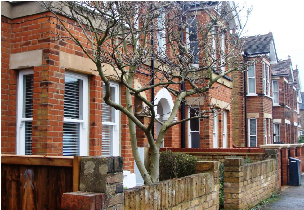
Picture 69. Good quality bay window detailing and recessed entrances, Fanshawe Street.
