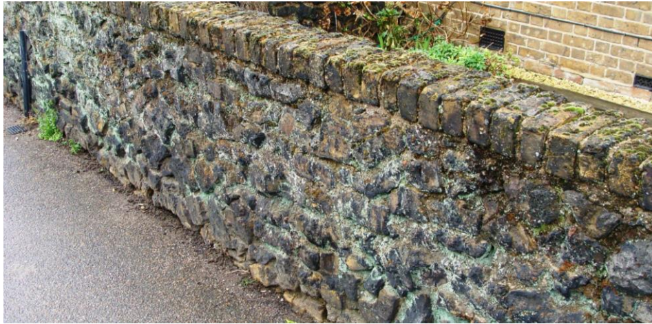
Picture 176. Unusual clinker wall construction to front of properties on Tamworth Road, worthy of retention and additional protection.
