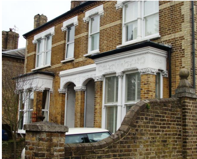
Picture 167. Decorative detailing to Nos. 51-53 Ware Road. Note boundary wall worthy of retention.
