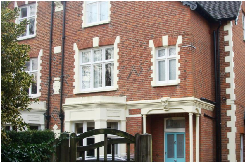
Picture 59. Good quality detailing that should be retained.
