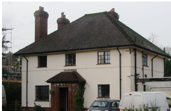
Picture 60. No. 17 Bengo Street. Some mid/late 20th century properties representative of their age add interest and diversity to the street scene.
