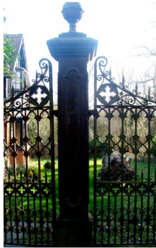
Picture 139. Access gates to Hertford Lodge (?)
