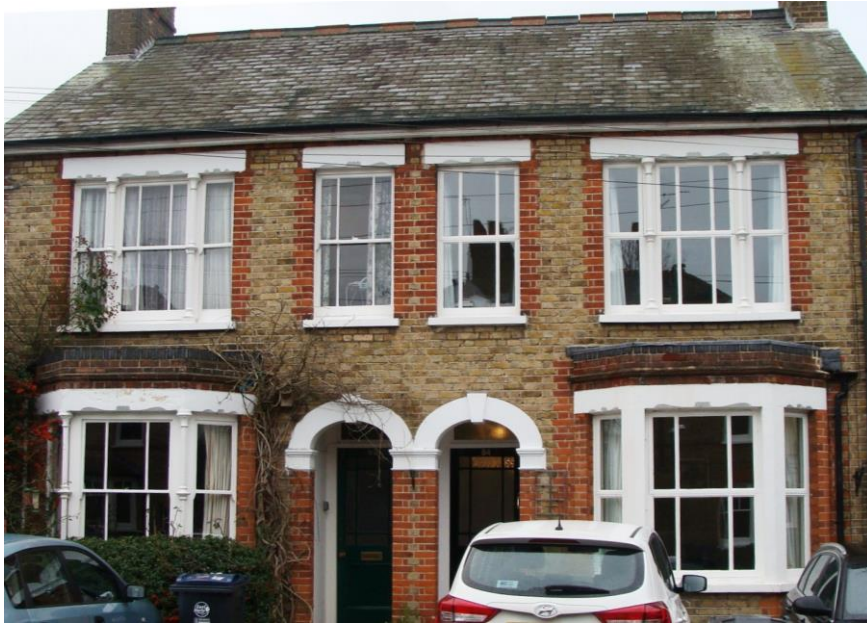
Picture 6. A better solution but one that could have been improved upon. The window surround detailing has been retained and this is important. It is particularly important that the recessed entrances have not been altered. The property on the left has early/ original windows whilst those on the right are heavier but nevertheless retain similar profiles to the originals. This is not an uncommon occurrence in the town.
