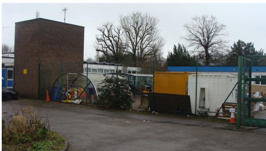
Picture 95. Part of Millmead school site detracts from quality of the conservation area and would benefit from comprehensive improvements.
