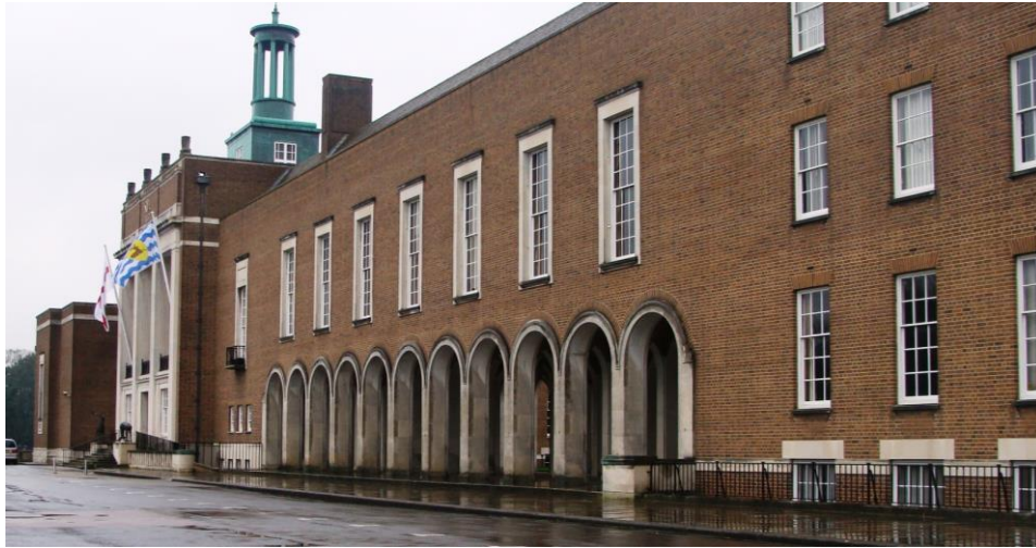
Picture 149. County Hall Architects James and Bywaters and Rowland Pierce. Design influenced by Swedish Romantic and Neo-classical architecture of the earlier 20th century and the work of Sir John Soane.
