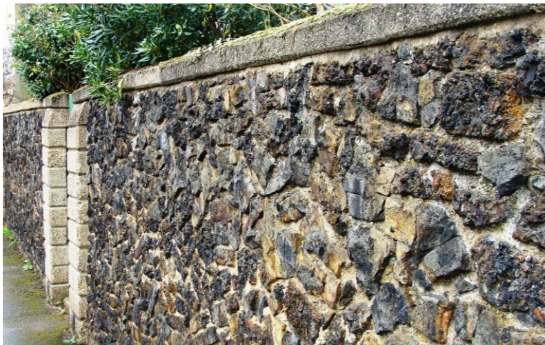
Picture 179. Unusual clinker wall of historic interest that adds variety to the local street scene and worthy of retention. Wall of similar construction on Tamworth Road.
