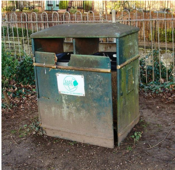
Pictures 41-42. Various detracting aspects of Millennium Sculpture area. Badly worn surfaces and shattered litter bin. This area is in real need of improvement, a view independently shared with the Hertford Urban Design Strategy.
