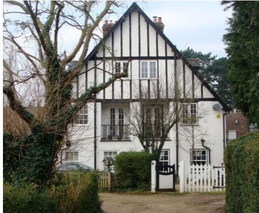
Picture 72. Nos.10-12 off Farquhar Street an interesting building probably dating from the 1920's.
