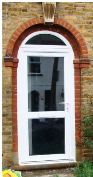
Picture 7. An example of where a recessed entrance has been enclosed. Compare the visual impact with those remaining open in the picture above.
