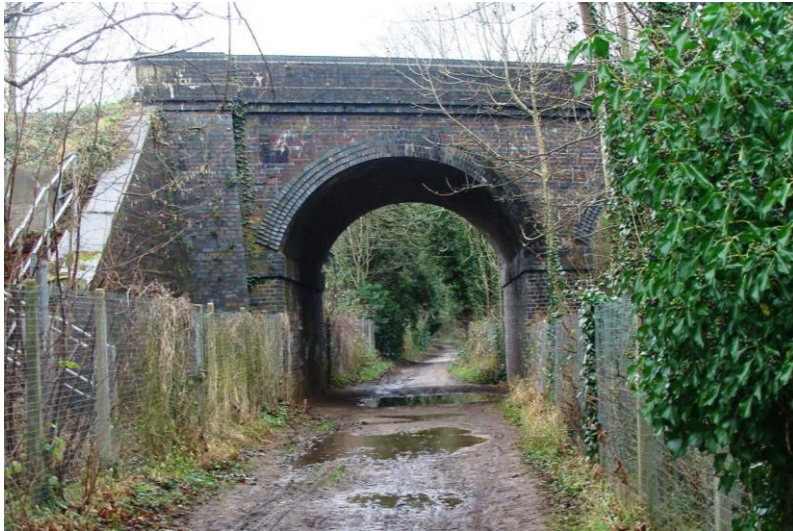
Picture 81. Bridge forming part of Enfield and Stevenage Loop Line.
