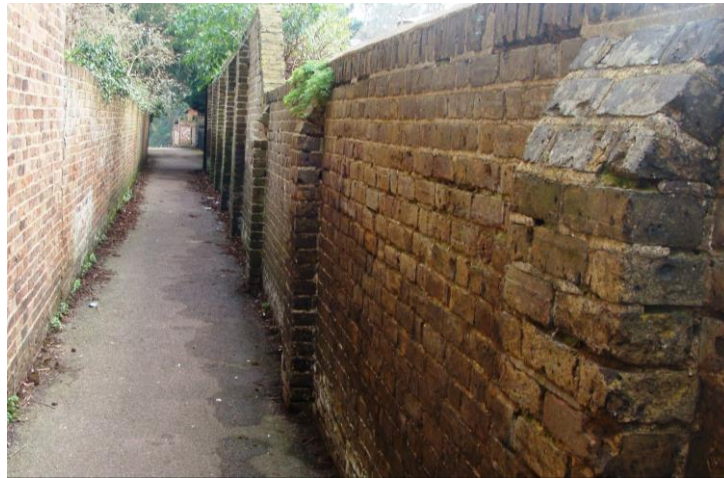
Picture 85. Walls enclosing public footpath 85.
