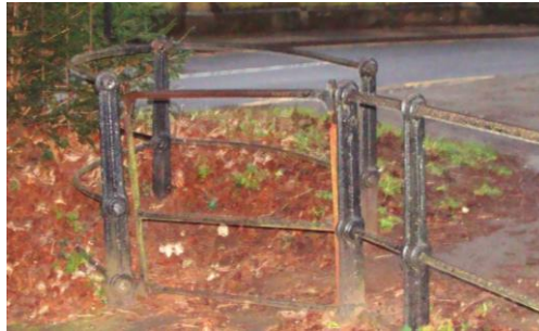
Picture 142. Boundary railing detail and entrance point to All Saints churchyard, south western corner.
