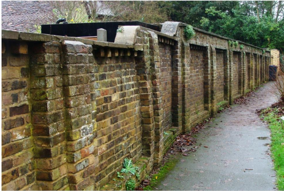
Picture 115. Prominent brick wall important to the quality of Warren Park Road.
