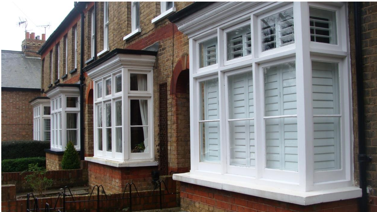
Picture 67. Nos. 15-21 Elton Road, part of a street that has retained many early features of quality.
