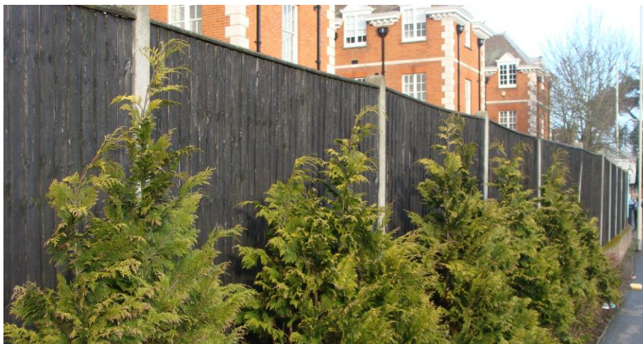
Picture 47. Inappropriate wooden fencing adjacent to concentration of listed buildings on Mill Road.
