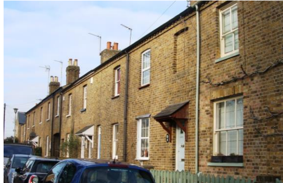
Picture 73. Balfour Street a typical 19th century street with some early porch detailing still remaining. Wouldn't it be nice to carefully replicate this detail above other entrances?
