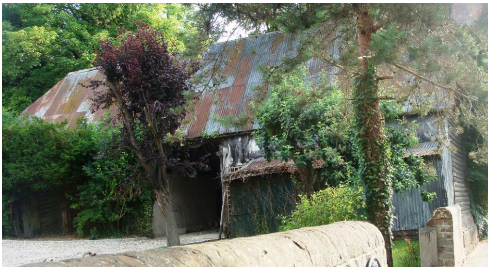
Picture 5. Grade II barn at Little Meadow, the corrugated roof was originally thatch. A thatch replacement roof would represent a significant gain. Potential grant assistance may be available. The building is on the Council's Heritage at Risk Register.
