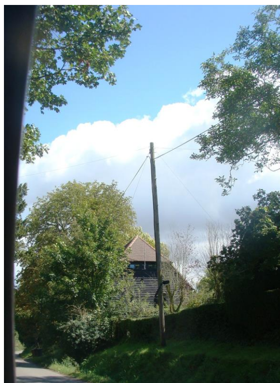
Picture 26. Within the conservation area there are a number of utility poles that detract from the quality of the environment to varying degrees. The Parish Council may wish to discuss the matter further with the appropriate company to see if there any opportunities to achieve selective improvements.
