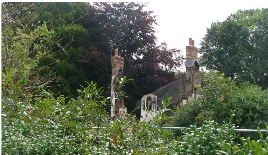
Picture 4. Hormead Cottage severely damaged by fire (December 2016). Discussions are taking place regarding its restoration.
