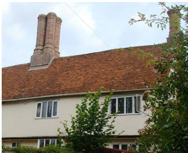
Picture2. Fine chimney detailing, The Old Rectory.
