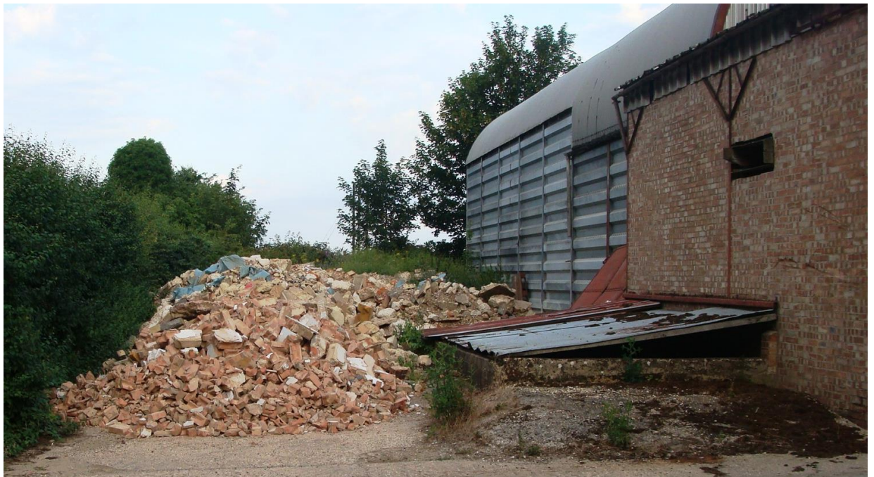
Picture 24. Brick rubble adjacent to the conservation area detracts. Hopefully discussions with the owner may secure improvements.
