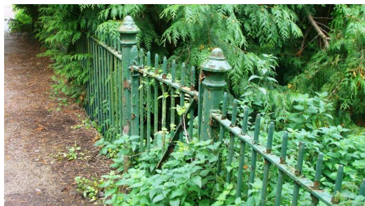
Picture 16. Good quality robust historic railings in need of minor repainting/refurbishment.
