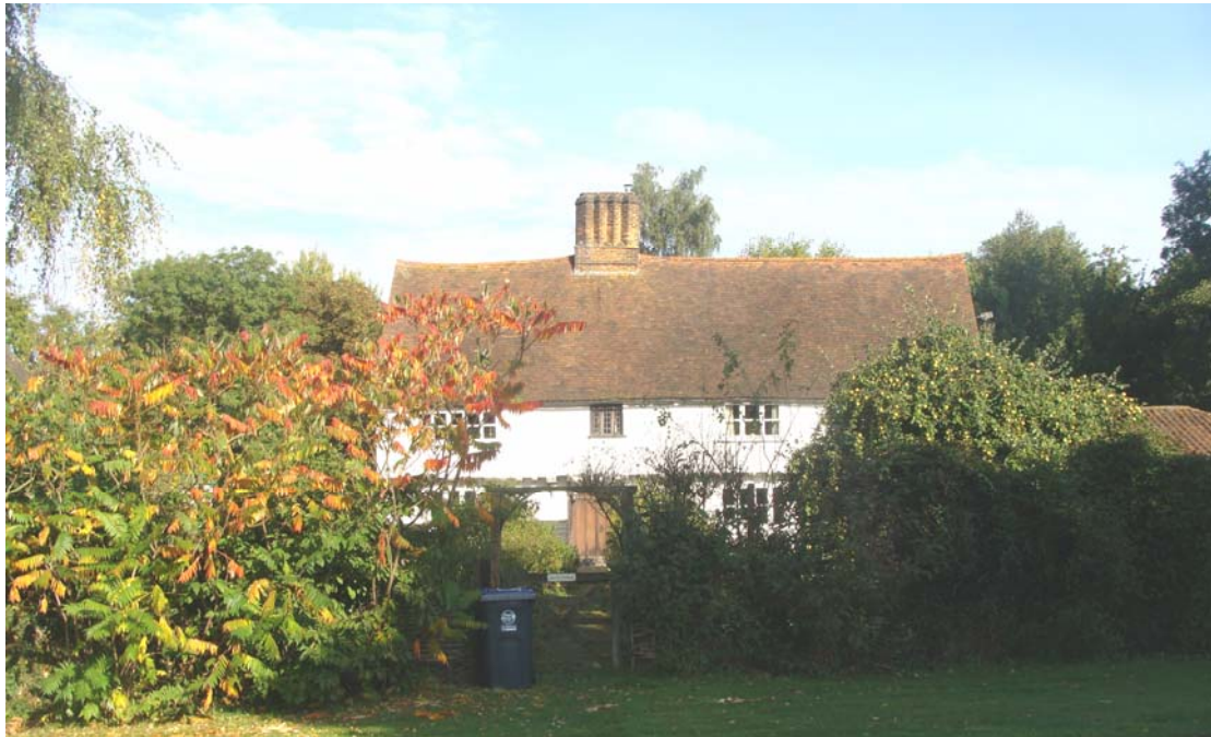
Picture 5 - Green Tye Farm House, an important 16 th century jettied building with old tiled roof and fine chimney detailing dating from the 17 th century.
