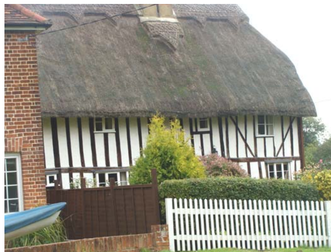
Picture 4 - Stuart Cottage, a thatched property dating from the 17 th century. Thatch is an important traditional material that should be retained.
