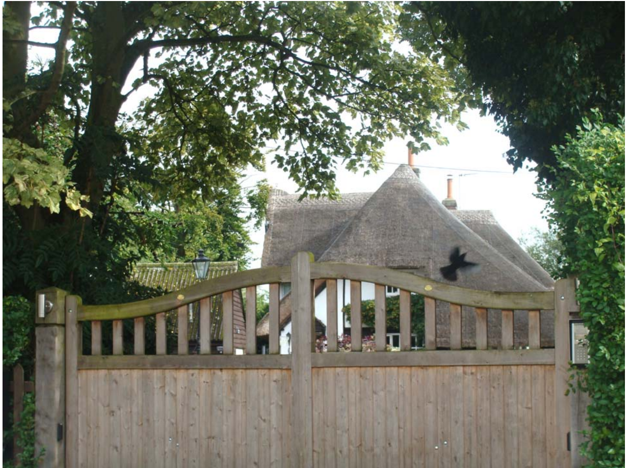
Picture 3 - Bulls Cottage, 16 th century in origin with thatched roof.
