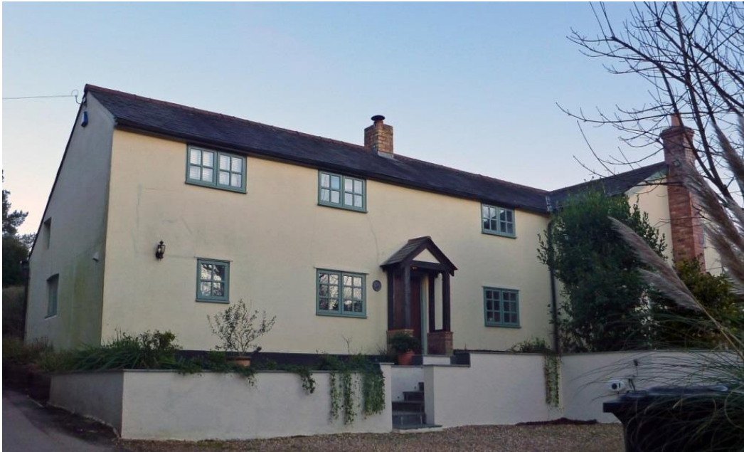
Fig. 36: Hill Cottage (south side) – Category 2 Late C19th detached house with plain rendered walls and a slate roof. Much altered.
