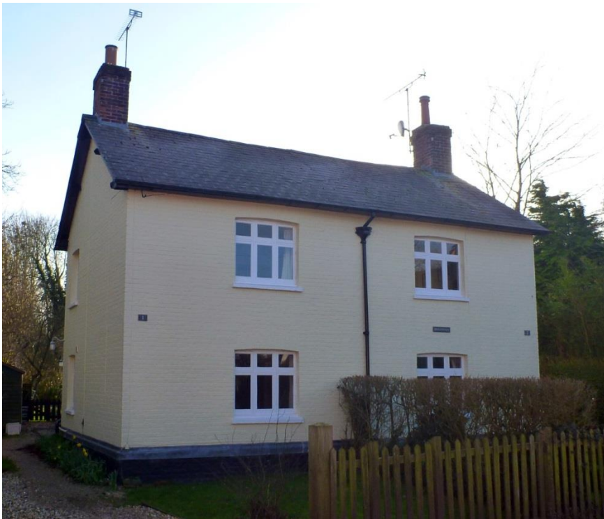
Fig. 33: Brick Cottages (south side) – Category 1 C19th pair of semi-detached houses in painted brick with a slate roof and two gable chimneys.
