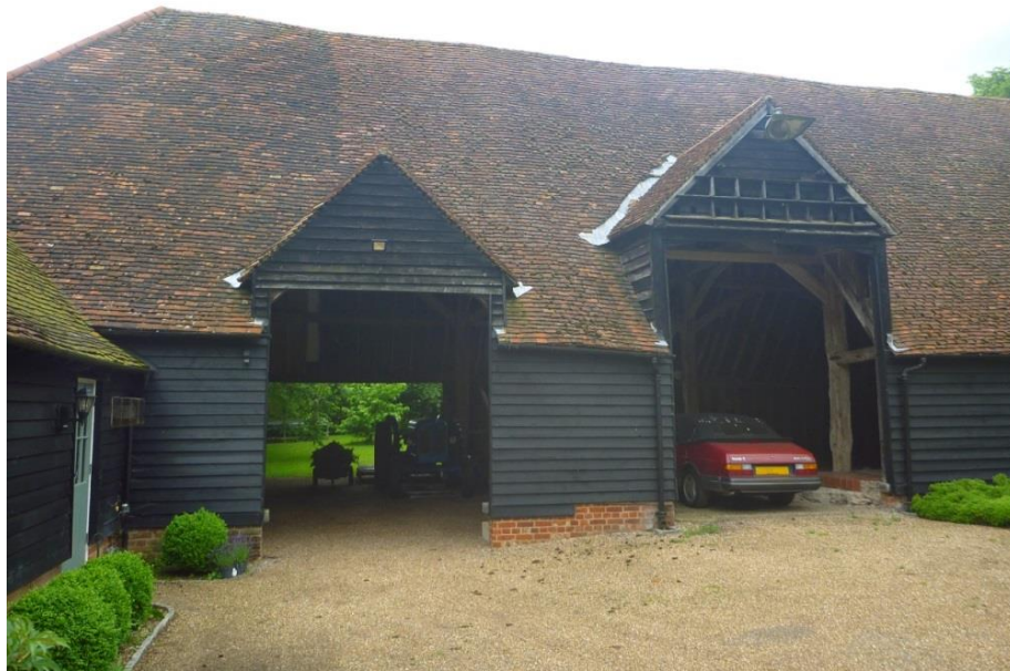
Fig. 9: Barn at Furneaux Pelham Hall
