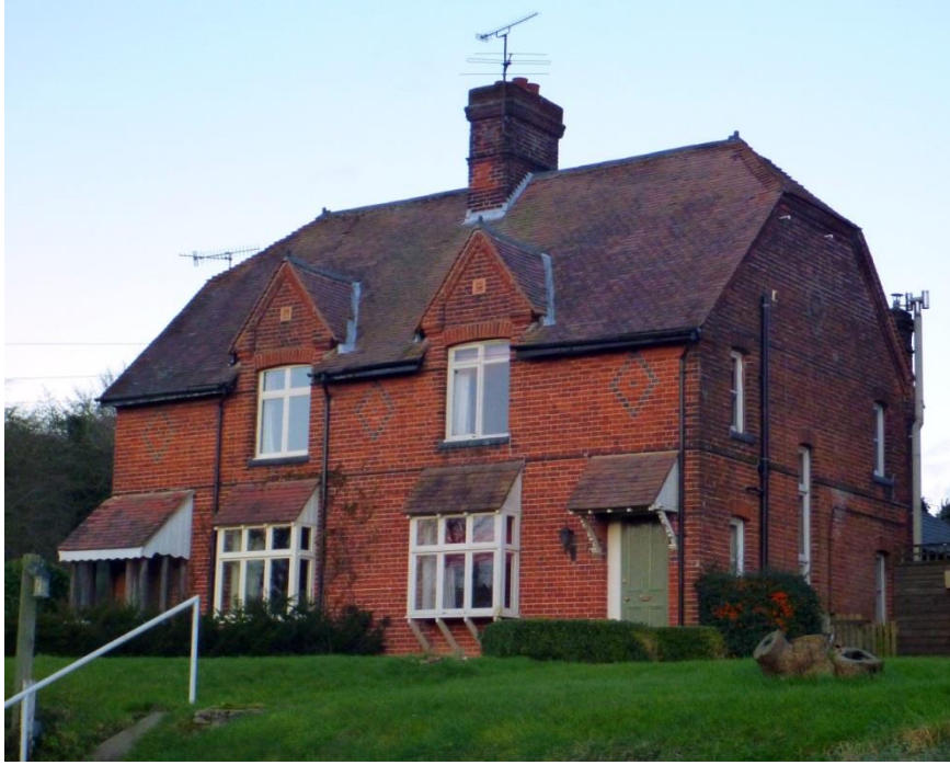
Fig. 48: 1 and 2 Lake Villas (east side) – Category 1
