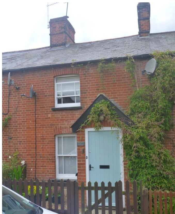
Fig. 43: Wrights Cottage (west side) – Category 1 Mid-terrace cottage shown on the C19th historic maps. Red brick and slate roof. Brick with slate roof modern porch. The windows should be retained.
