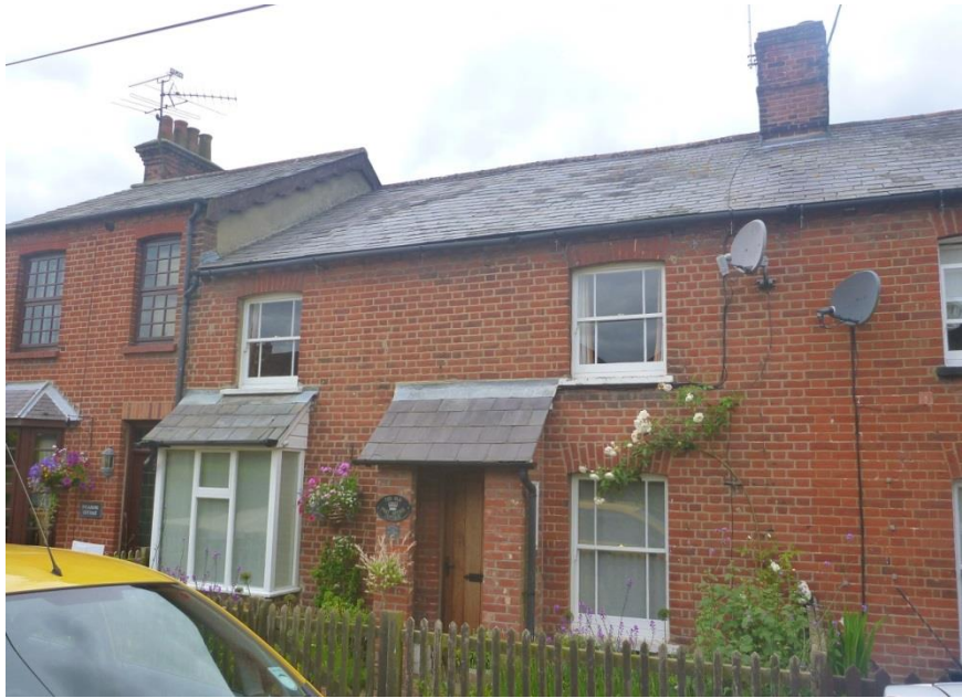
Fig. 42: The Old Post Office (west side) – Category 1 Mid-terrace cottage shown on the C19th historic maps. Red brick and slate roof. Brick with slate roof modern porch. The windows should be retained. Later square bay (LHS) may date from when this cottage contained the village post office.
