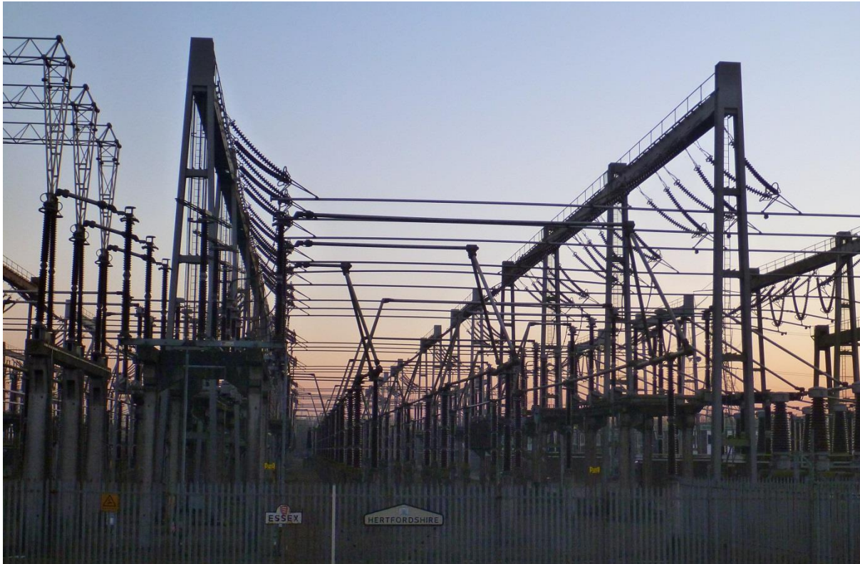
Fig 10: The Herts and Essex Electrical Transfer Station to the south of the Conservation Area has harmed its rural open setting.
