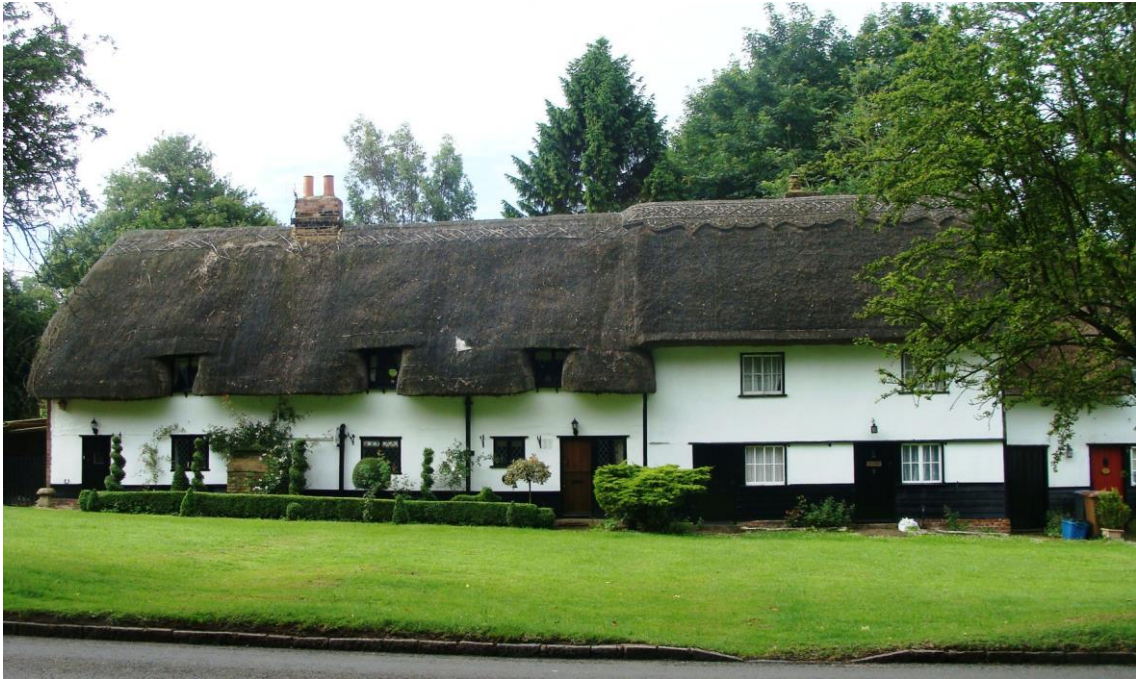
Picture 6. Home Close Cottages, picturesque with steeply sloping thatched roof and eyebrow dormers.
