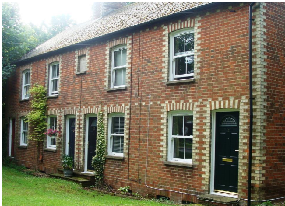
Picture 17. Nos. 1-4 Victoria Cottages - a prominent and pleasing terrace dating from the late 19th century in the centre of the conservation area and largely unspoilt.
