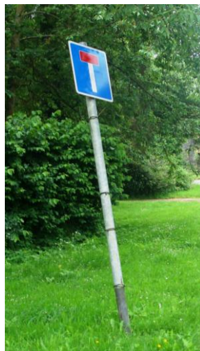
Picture 47. No entry sign Warren Lane needs re erecting.
