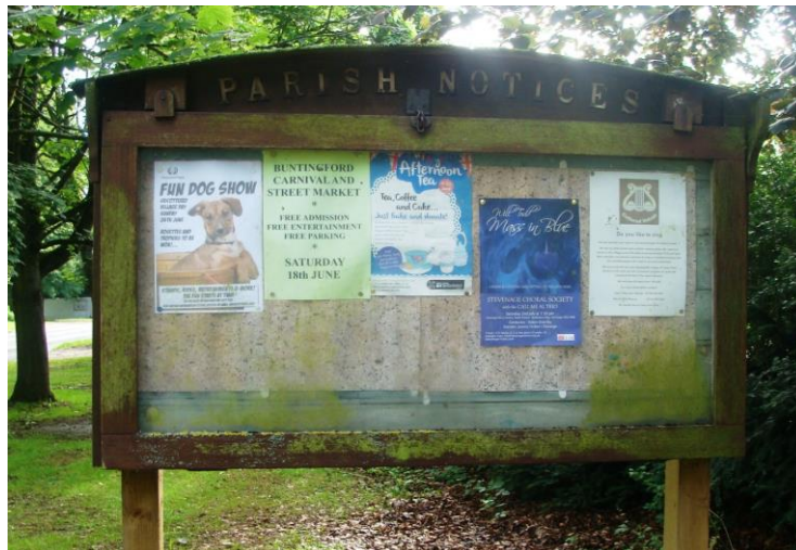
Picture 45. Improvements to the notice board would be beneficial.
