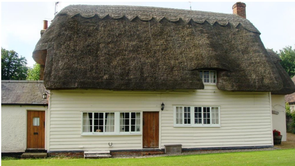
Picture 7. The former Bell PH. One of a number of important listed thatched properties in Cottered.
