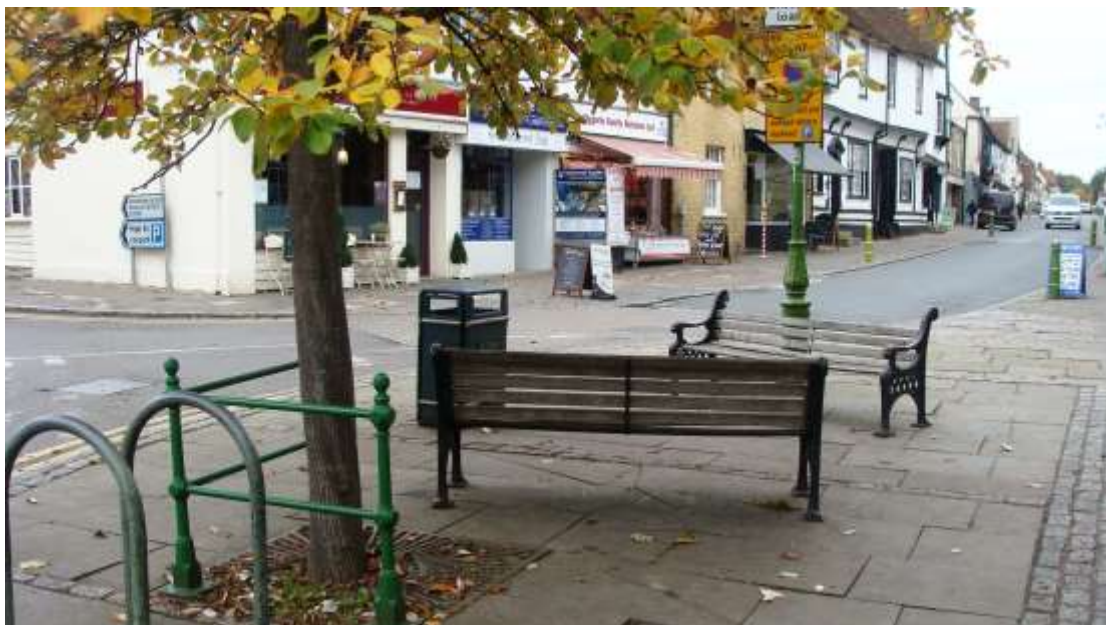
Picture 63. Minimum works involve repairs to one of the pair of seats.
