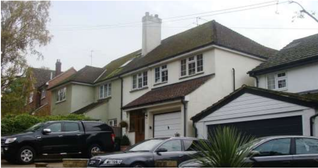
Picture 72. Nos. 2 - 6 and Layston House, The Causeway, now excluded from the Conservation Area.
