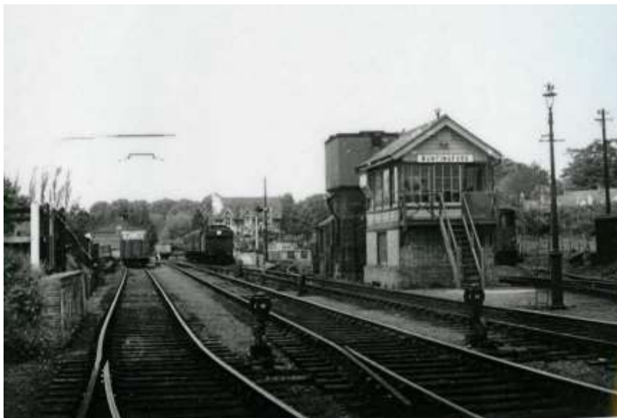
Picture 4. The railway station and branch line (1863-1965, freight). Now Fairfield Estate area. Reproduced from the collection of the late Philip W. Plumb and The Buntingford in Old Photographs Facebook page.
