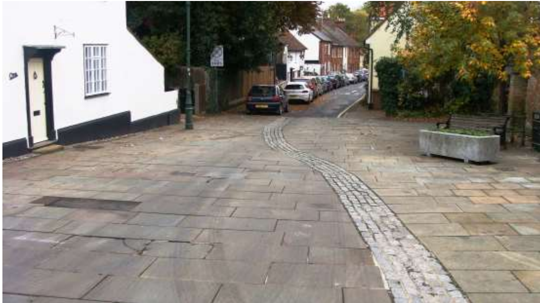
Picture 49. 'Shared space' junction High Street and Church Street. In the author's opinion it could perhaps be improved to make it more vibrant.
