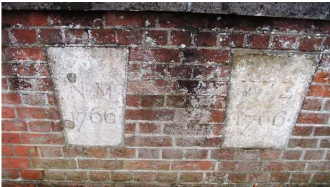
Picture 43. Historic plaques on bridge presumed to have formed part of an earlier bridge structure.
