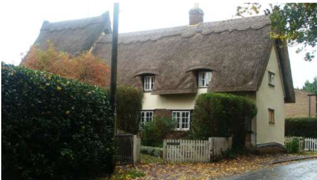
Picture 15. One of only two thatched properties in the Conservation Area.
