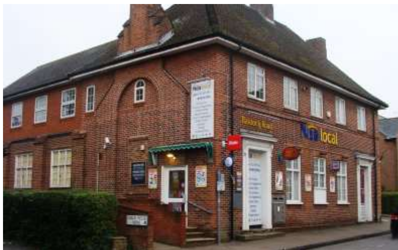
Picture 28. Local Nisa store. A robust mid 20th century property, a good example of its period and worthy of retention. Shows on OS mapping as being a Post Office for which purpose it may have originally been built. Some modest rationalisation of signage would be of considerable benefit to the street scene.
