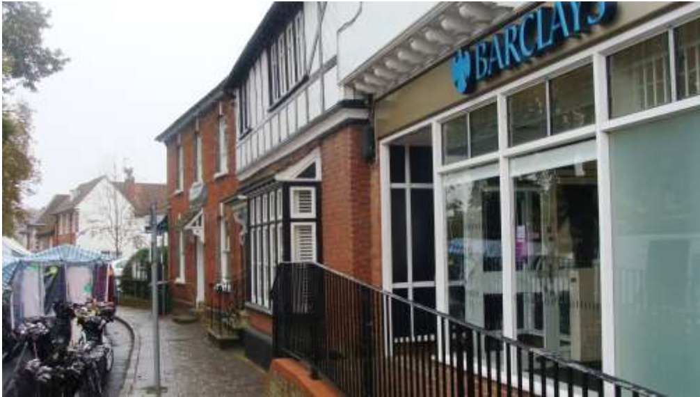
Picture 27. Group of properties displaying good quality architectural detailing which positively contribute to the townscape and which should be retained.
