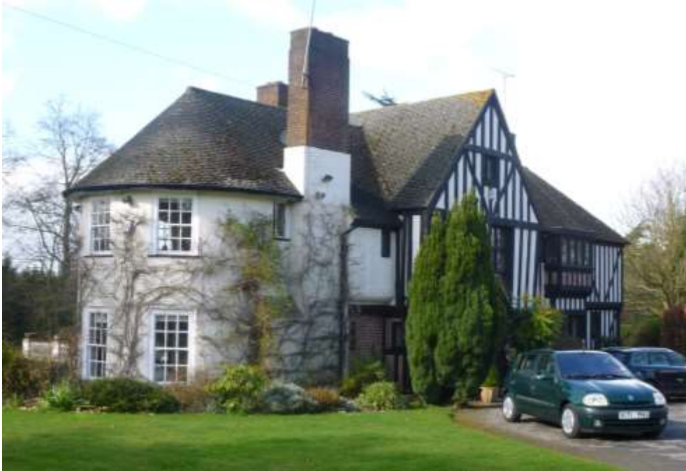
Picture 15. Sweetings - the curved elevation is to original design by Clough Williams Ellis but the 'Elizabethan' façade is a later addition dating from the 1980's. Photo reproduced courtesy of John Lambie.
