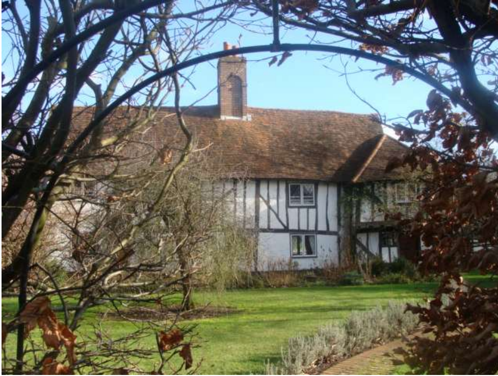
Picture 4 - Bentleys a fine grade II listed building dating from the 15th century.
