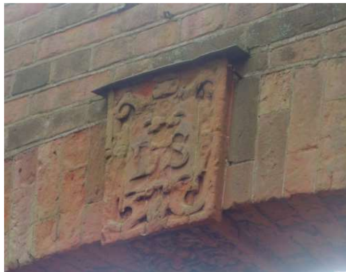
Pictures 23 and 24. Prominent garden walls of considerable architectural merit and historic importance south east of Fanshaws mansion and in good condition.
