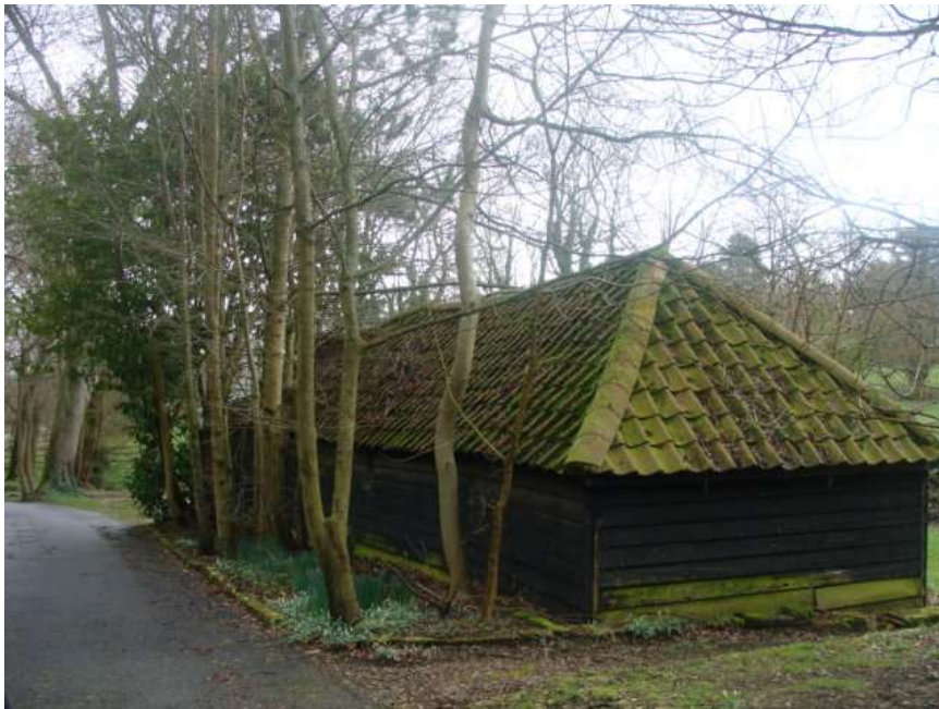
Picture 22. Simple barn dating from late 19th/early 20th century most worthy of retention.
