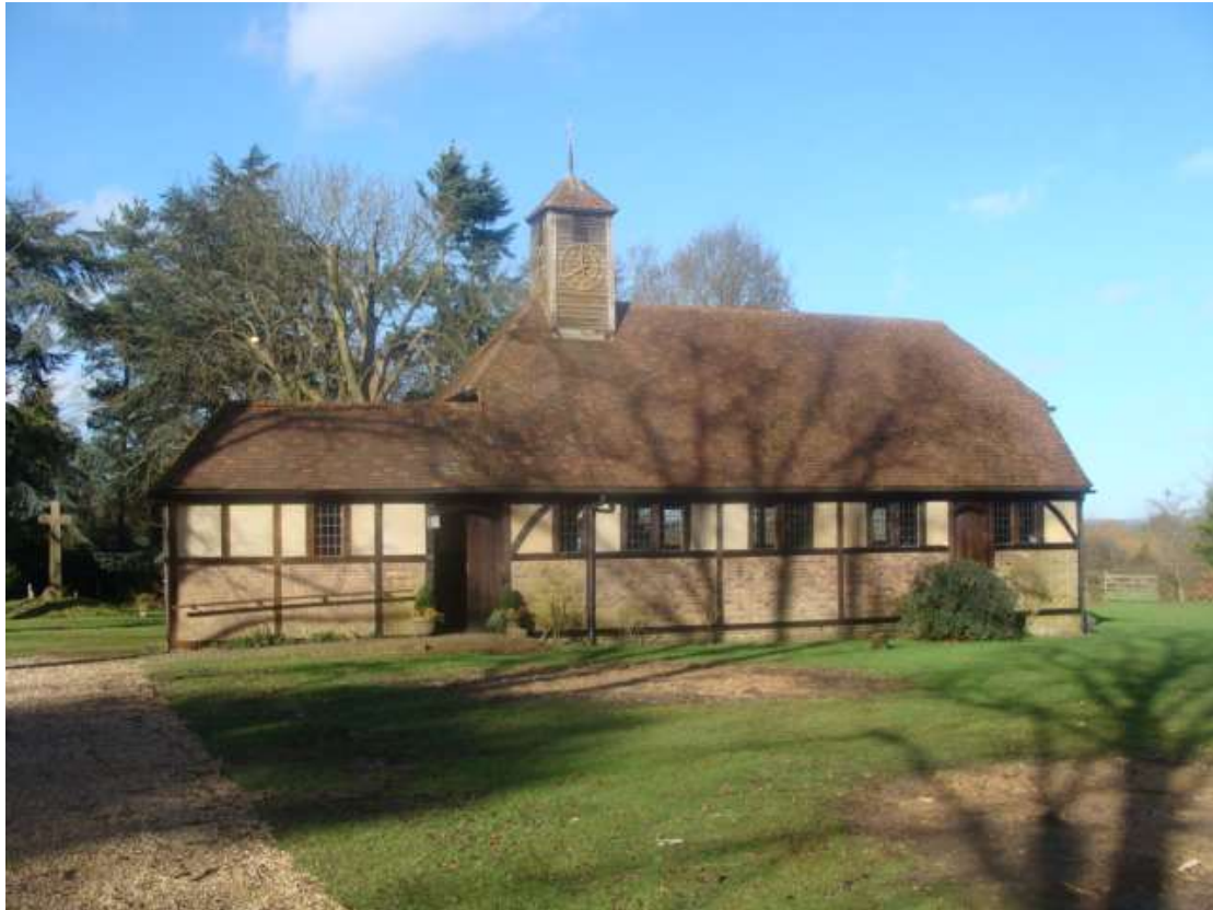
Picture 16. Chapel of the Holy Cross and Saint Alban built in the early 1930 by Rattee and Kett. A charming structure well detailed externally and internally.
