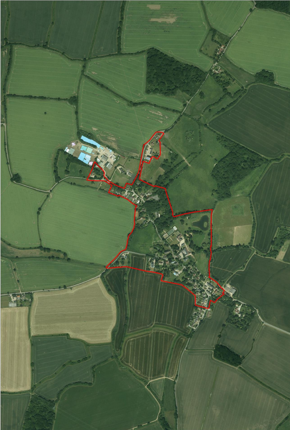
Fig. 1: Aerial Photograph from 2015
