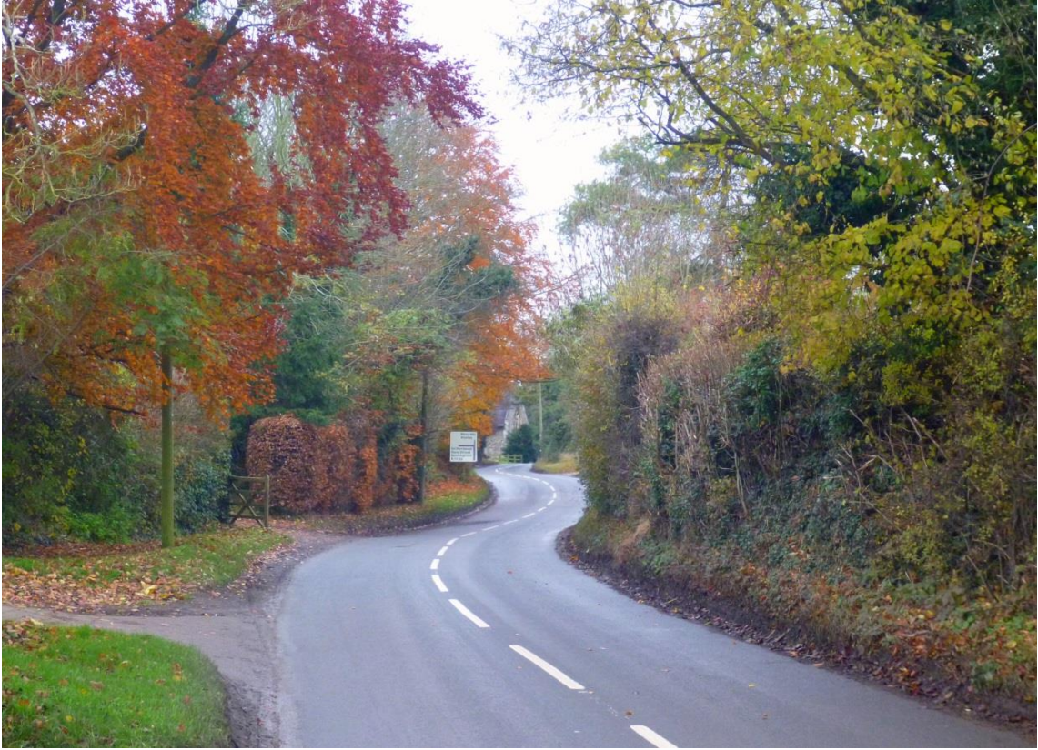
Fig. 58: View looking north along Pump Hill.
