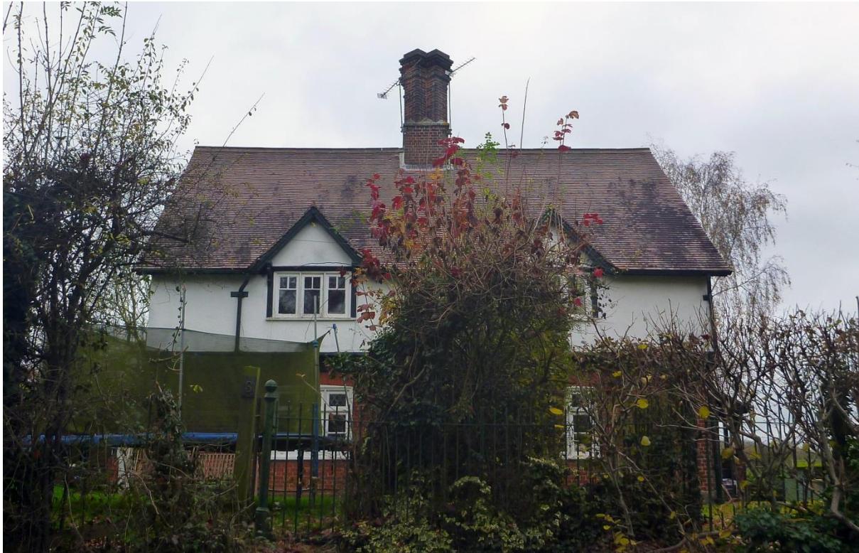
Fig. 38: 3 and 4 Pump Hill, built in the first decade of the C20th
