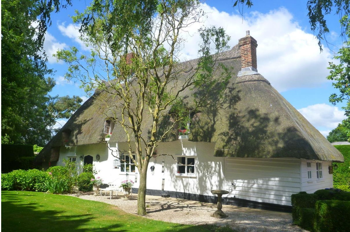
Fig. 14: Bridge Cottage. This is C16th or earlier, and is timber-framed, rendered and part weather-boarded, under a thatched roof. It is of one storey and attics.
