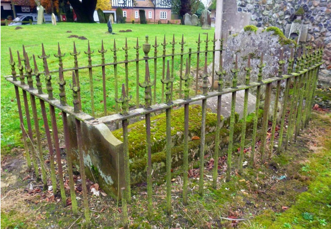
Fig. 43: The railings around a grave at the eastern end of the Church
