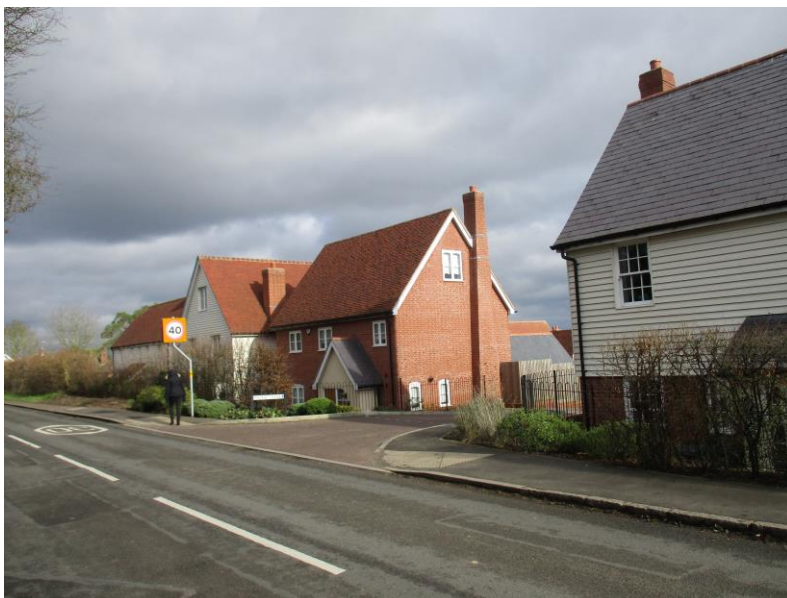
Neutral modern development with floor levels that do not successfully address the street.
