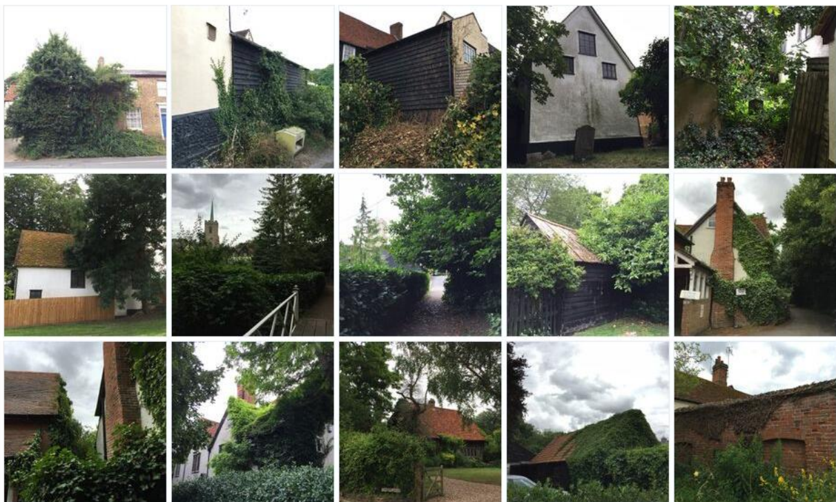
Overgrowth of vegetation
