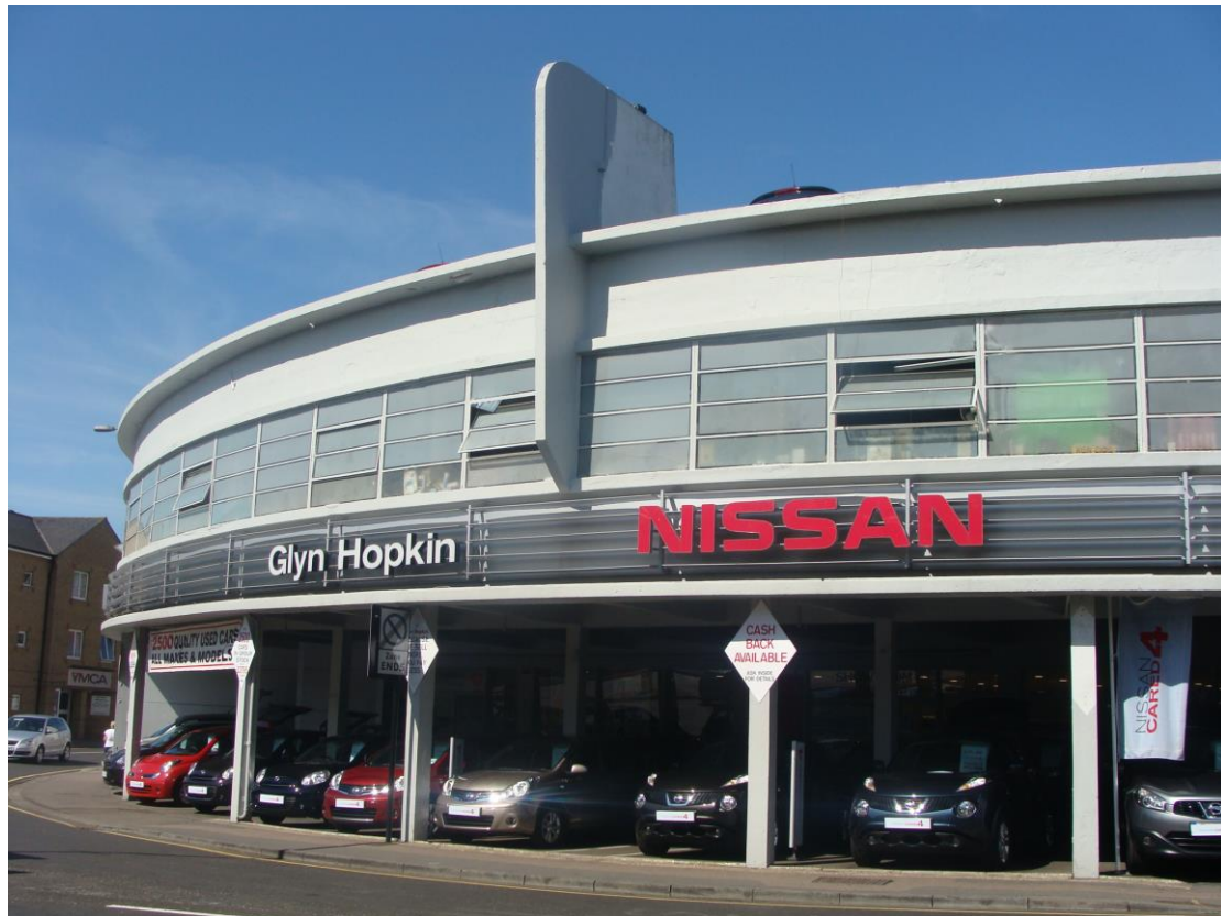
Picture 80. Attractive early/mid 20 th century building of unusual design and quality on a prominent corner plot.
