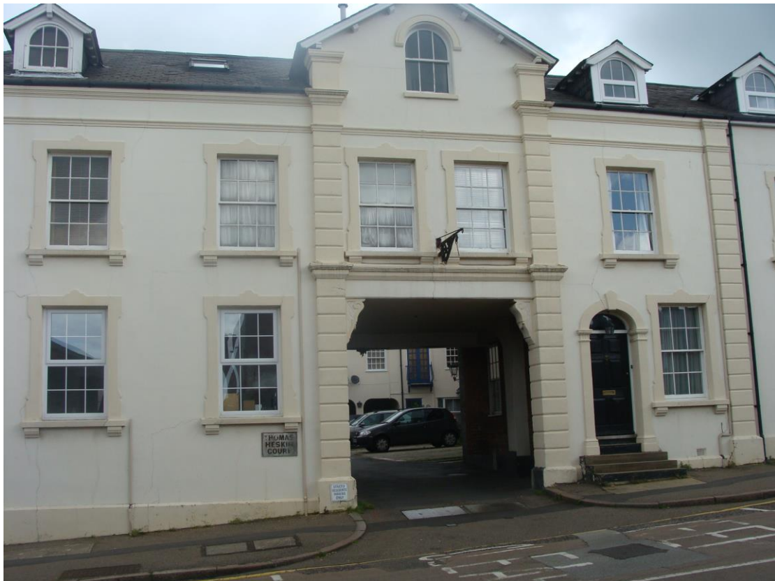
Picture 26. Thomas Heskin Court, an important unlisted building on a prominent corner of London Road and Station Road.
