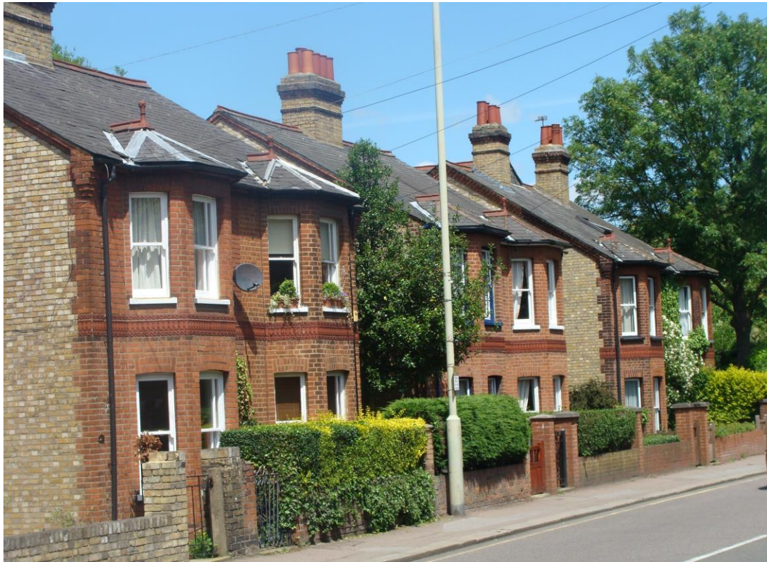
Picture 25. Nos. 25-35 Stansted Road. Repetitive architectural detailing adds to their individual quality and quality as a group.
