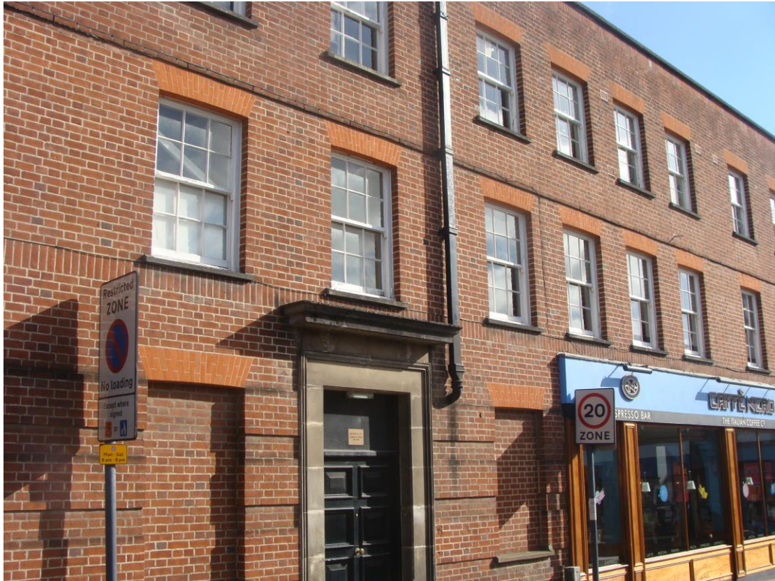
Picture 90. Café Nero, corner of Apton Road and Potter Street. Interpreted as dating from early/mid 20 th century. Its simplicity and repetitive rhythm of windows contributes to its visual success.
