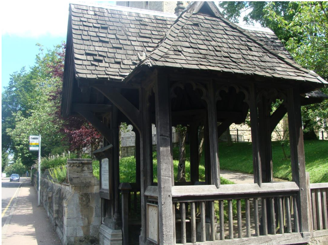
Picture 20. Lych Gate at Church of All Saints, of oak construction. Shingle roof and old bench seats,
