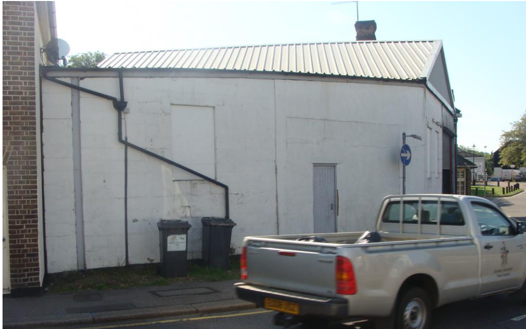
Picture 57. One of several poor quality buildings in and around the Mill area. Such buildings provide employment but are visually damaging to this part of the town centre.
