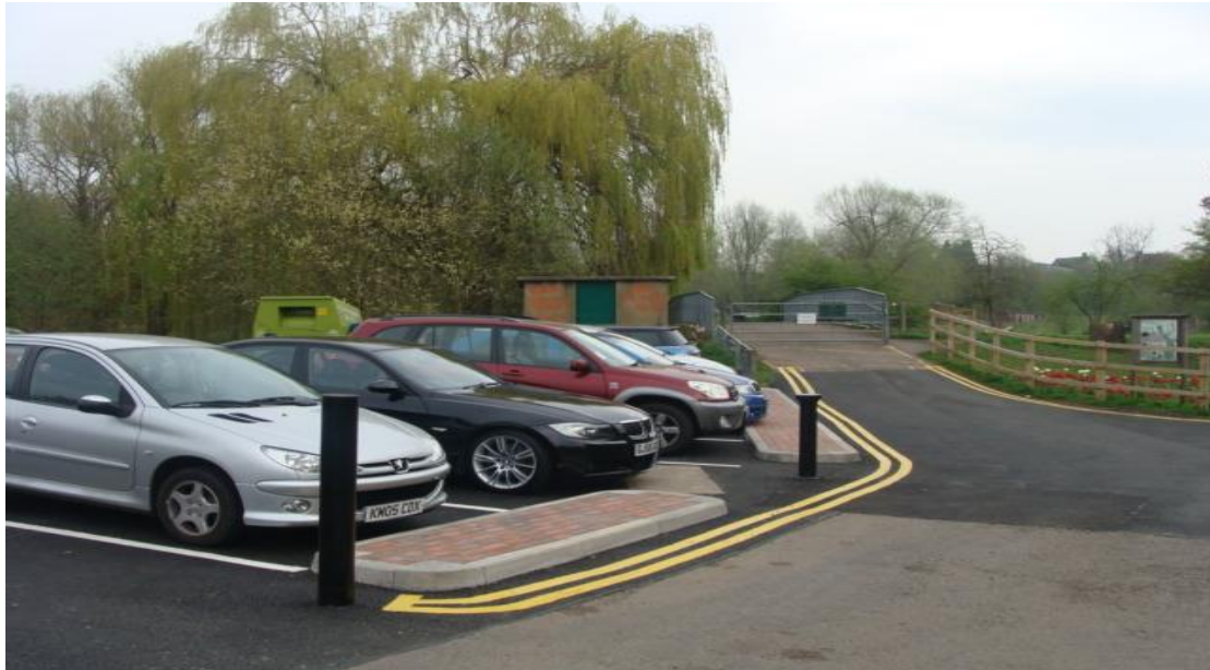
Picture 56. The metal barriers of previous picture now replaced with raised surface and bollards.
