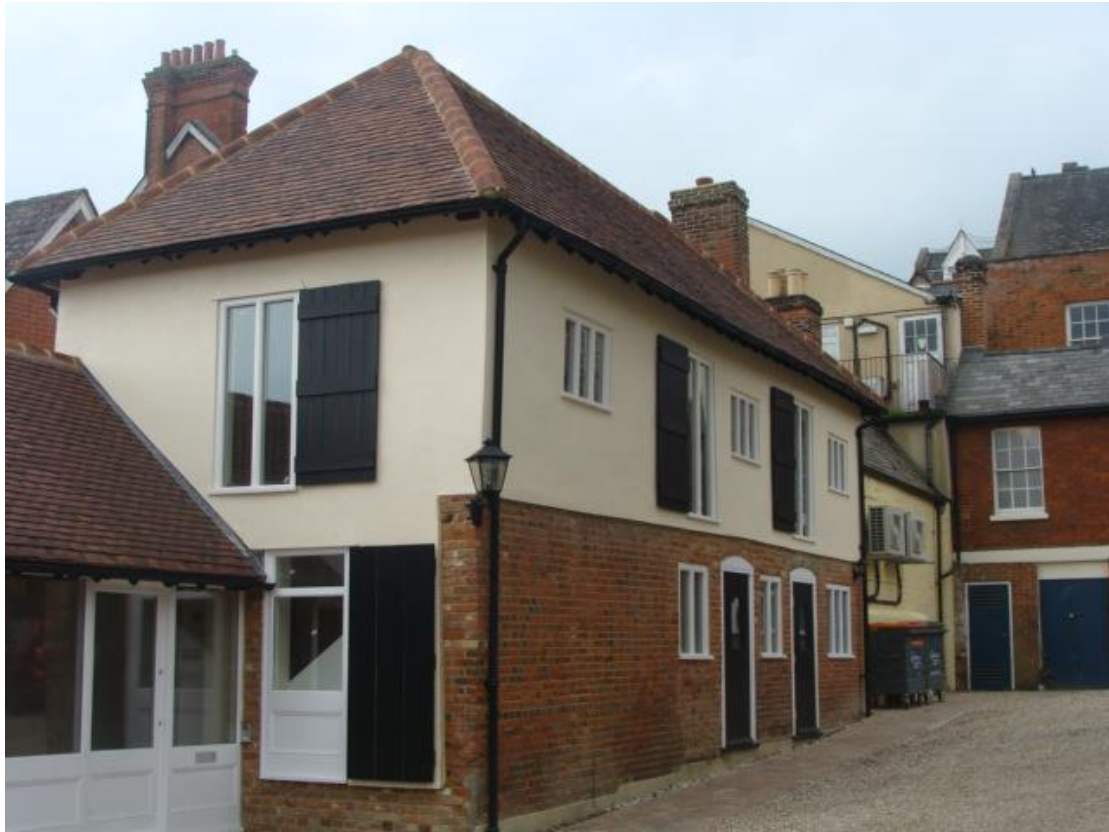
Picture 79. The same building as above, now restored.
