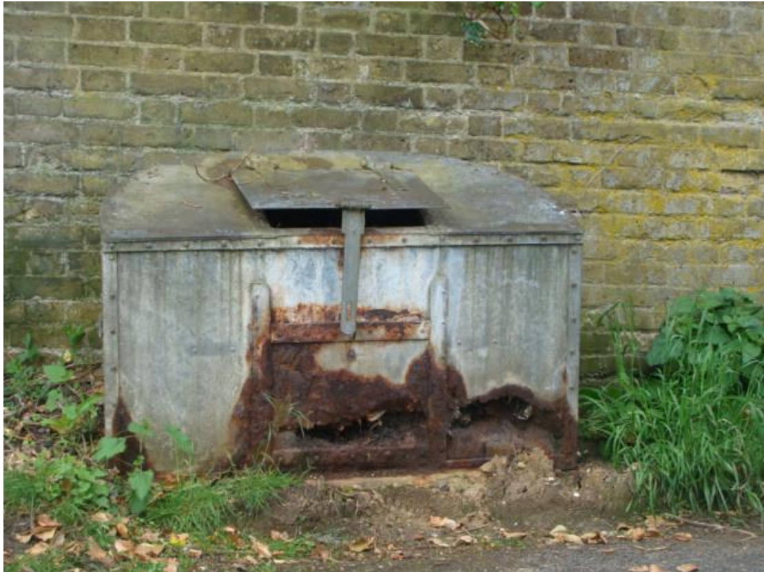
Picture 99. Redundant salt bin, Windhill Old Road which is most unattractive.
