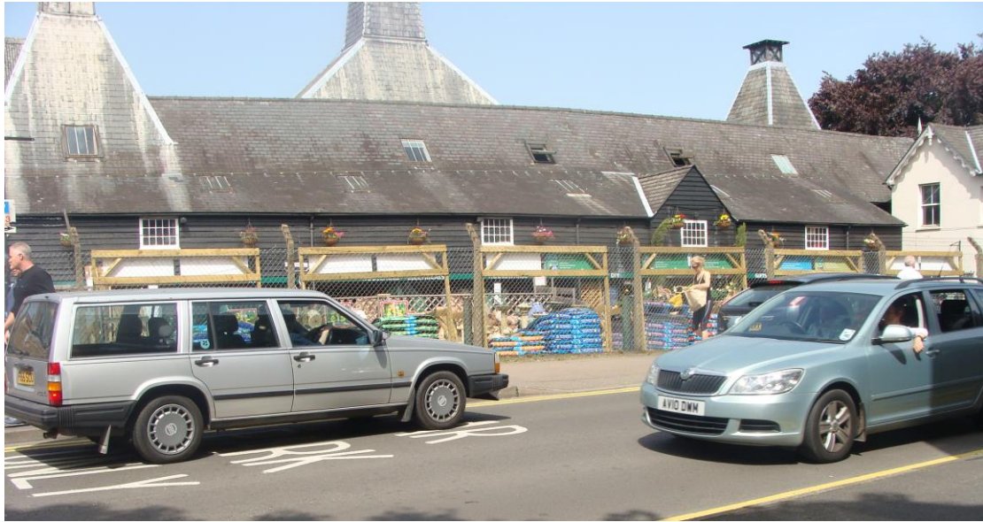
Picture 100. Boundary fence to Coopers of Stortford and Rivetts, Old River Lane detracts in an important town centre location.
