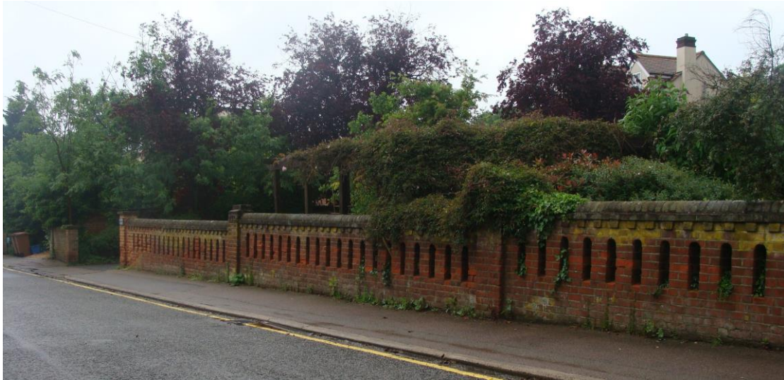
Picture 15. Distinctive boundary wall at Chantry Road, part of which is proposed for inclusion within an extended Conservation Area.
