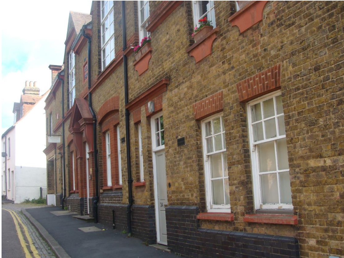
Picture 91. Nos. 24-26A, The Old Courthouse, Church Street; part of a varied group displaying different architectural detailing, massing and scales, particularly attractive in this narrow street with different profiles and gradients.
