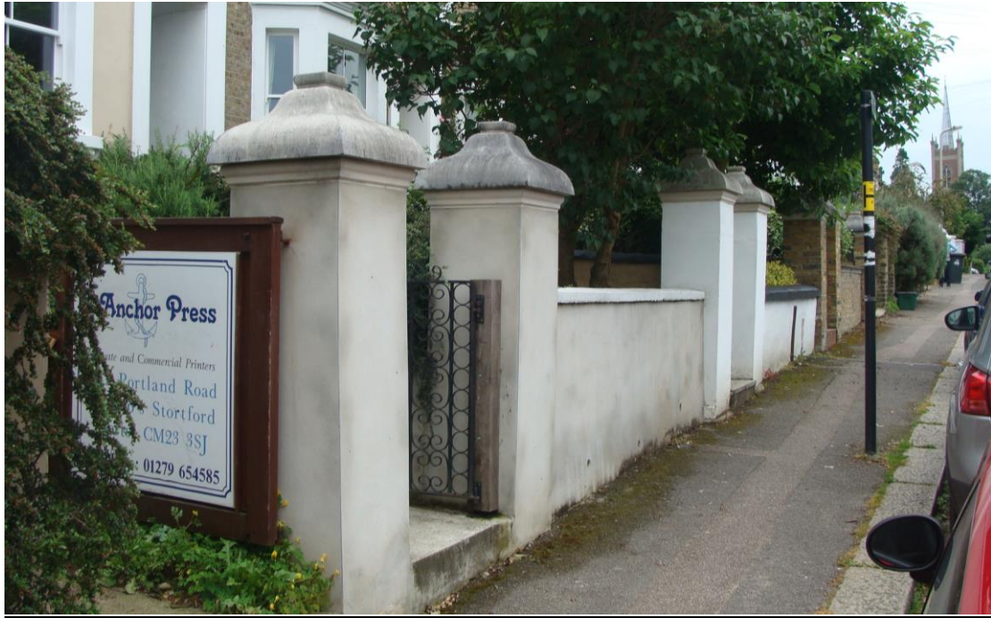
Picture 71. Representative front wall and pillar detailing to nos. 42- 44 Portland Road. Similar simple detailing would likely have been repeated along the frontage of these terrace blocks. The sign for Anchor Press is redundant and would benefit by being removed.
