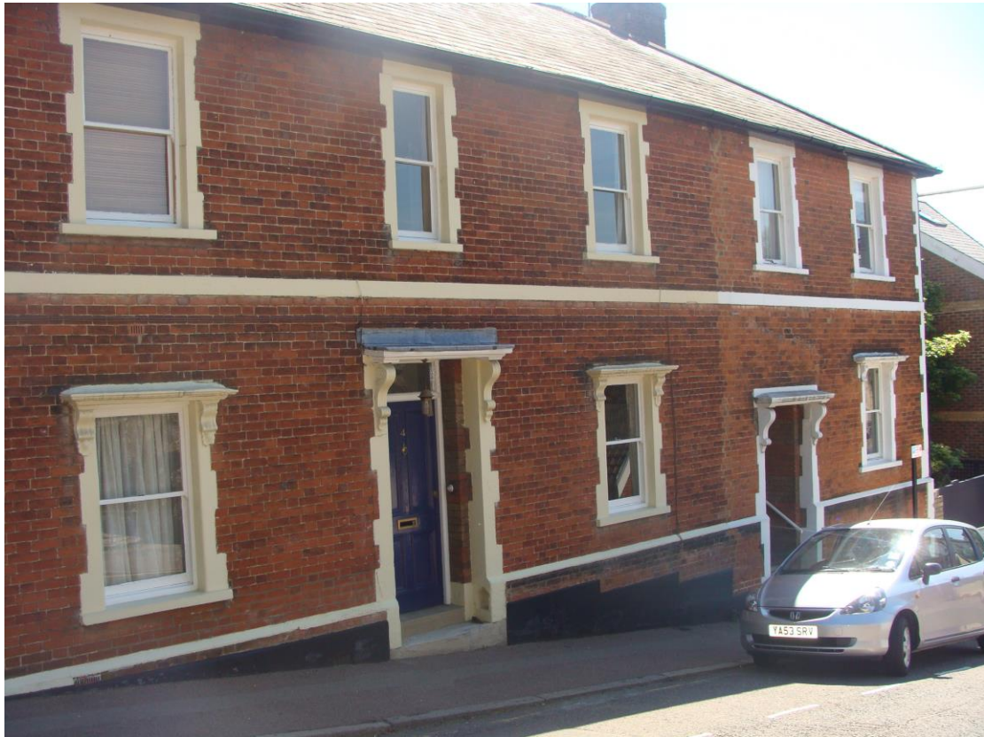
Picture 81. Nos. 2-4 Chantry Road. 19 th century pair of non listed houses with decorative window and door surrounds, worthy of retention.
