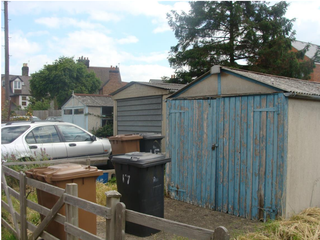
Picture 37. Garaging of a temporary nature associated with Crown Terrace adjacent to EHDC surface car park.
