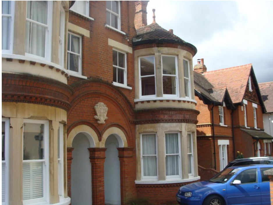
Picture 30. Nos.32-34 Grange Road, part of the street now included in the extended Conservation Area.
