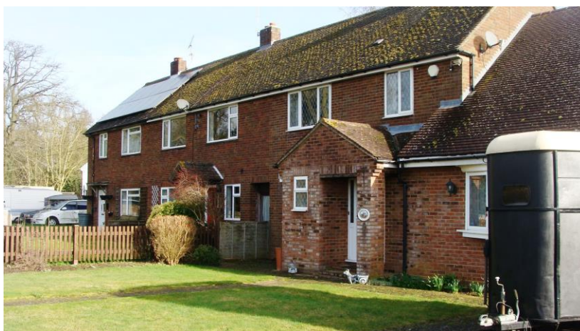
Picture 34. Nos. 3-5 Astonbury Farm Cottages. The original simple lines of these 20th century properties in a peripheral location have been visually compromised by extensions and a large area of solar panels.
