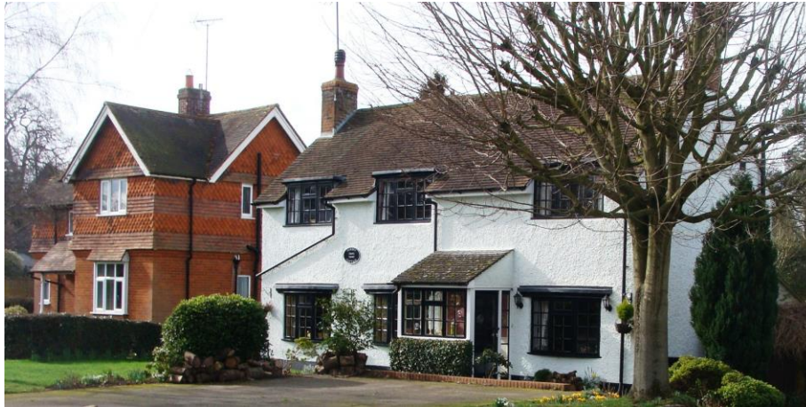
Picture 13. Garden Cottage- a simple elevation which together with adjacent Farm Cottage, makes a worthwhile visual contribution to the street scene.
