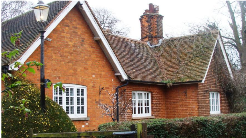
Picture10. The Lodge a pleasantly detailed lodge building which dates from the early 20th century.
