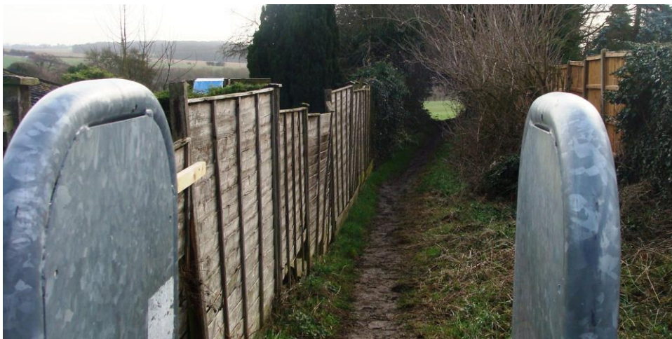
Picture 33. Broken fencing adjacent to footpath detracts. For information the metal guards prevent access by quad bikes.
