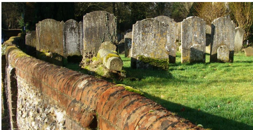
Picture 20. Prominent brick wall to churchyard frontage.
