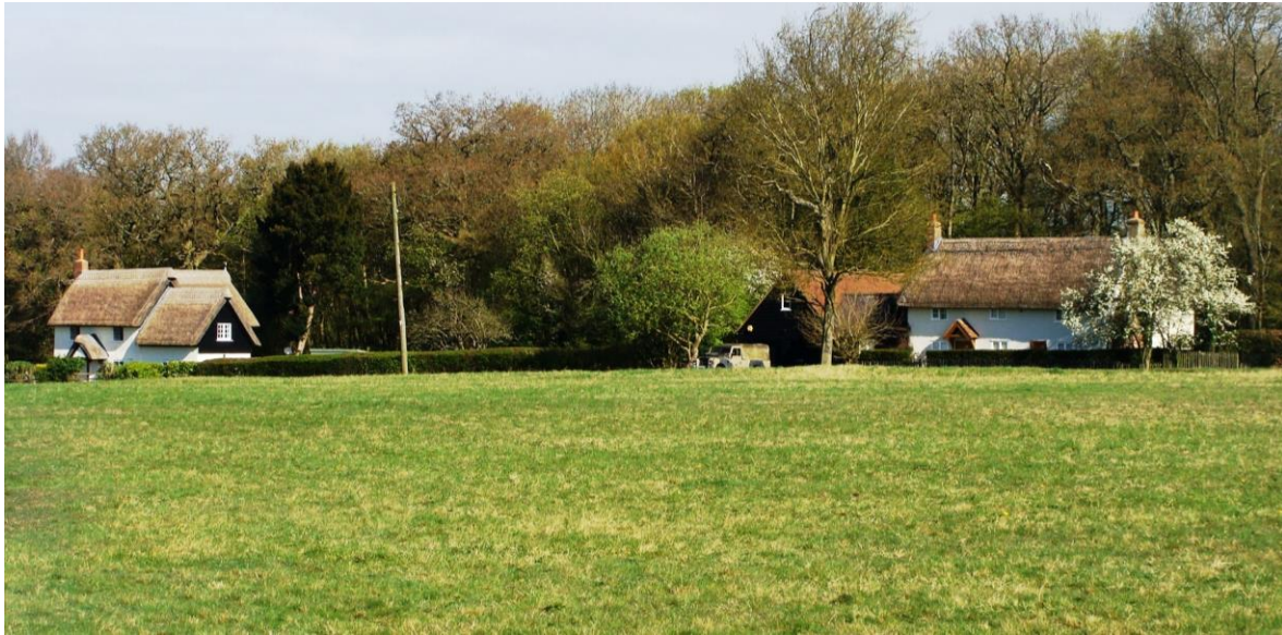
Picture 28. Two high quality listed buildings which together with the wood behind frame the extensive green when viewed from the south. Woodside Cottage on the left is described as having a pantiled roof at time of entry??
