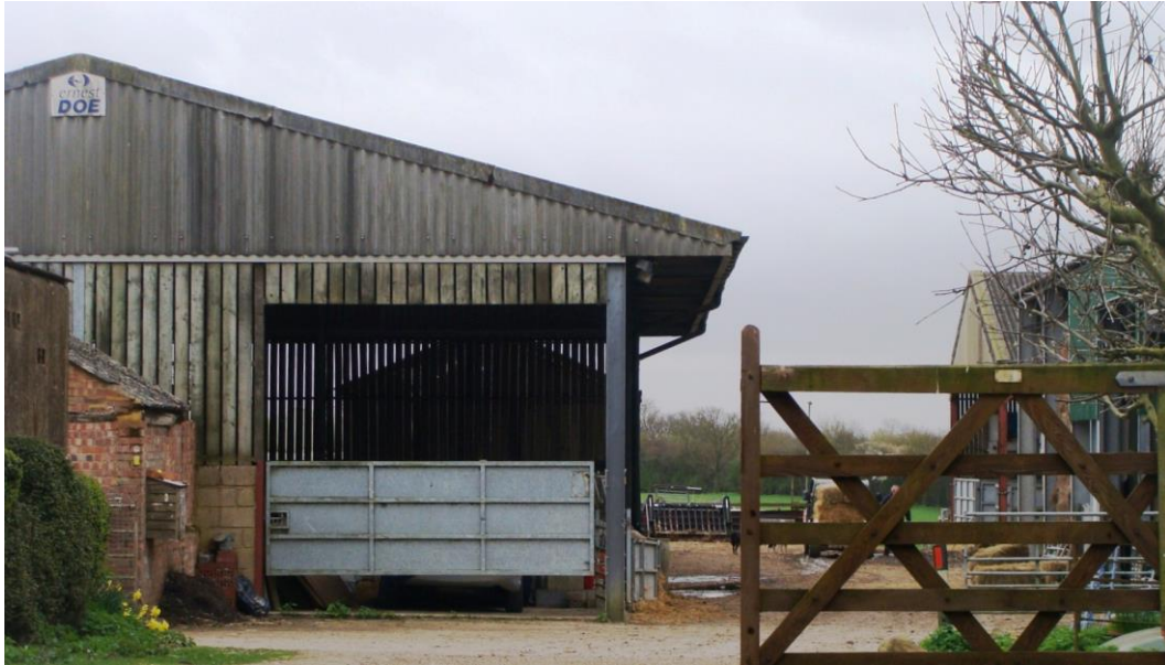
Picture 54. Modern agricultural buildings of no architectural merit or historic interest to rear of Highbury Farm and now excluded from the conservation area.
