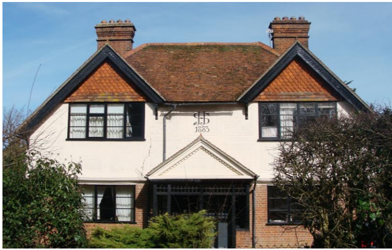
Picture 8. Nos. 1-2 Church End. A pair of symmetrical late 19th century properties with distinctive roof and chimney details.
