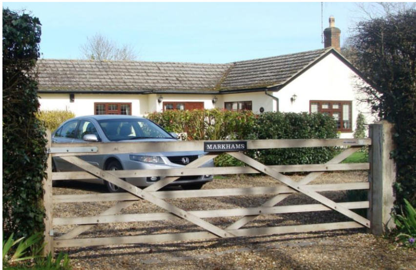
Picture 23. Markham's a bungalow from the 20th century on the edge of the conservation area is of insufficient architectural or historic interest to warrant continued inclusion in the conservation area.
