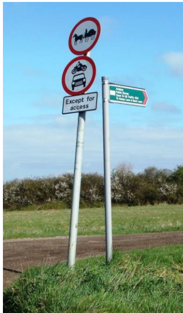
Picture 33. Pole out of correct vertical alignment detracts. Would it be possible to combine all necessary information on one pole?
